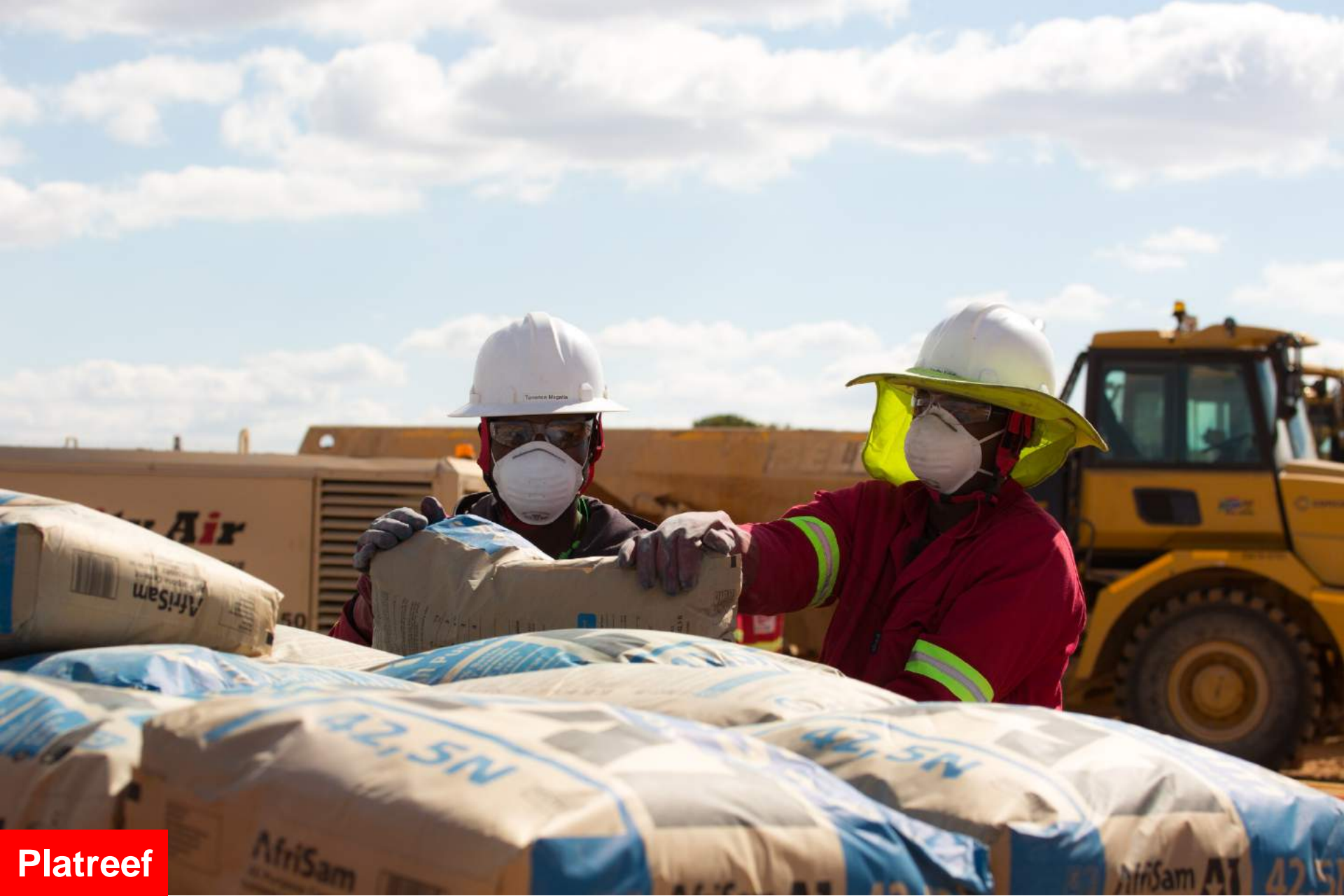
Platreef contract employees preparing for grouting of the side walls at Shaft 2 box cut.
