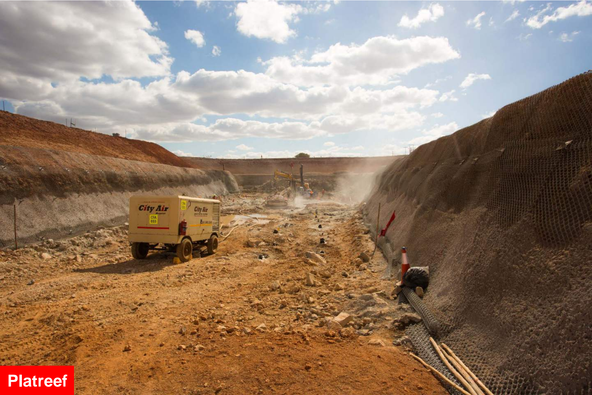
Drilling blast holes at the box cut for Shaft 2.
