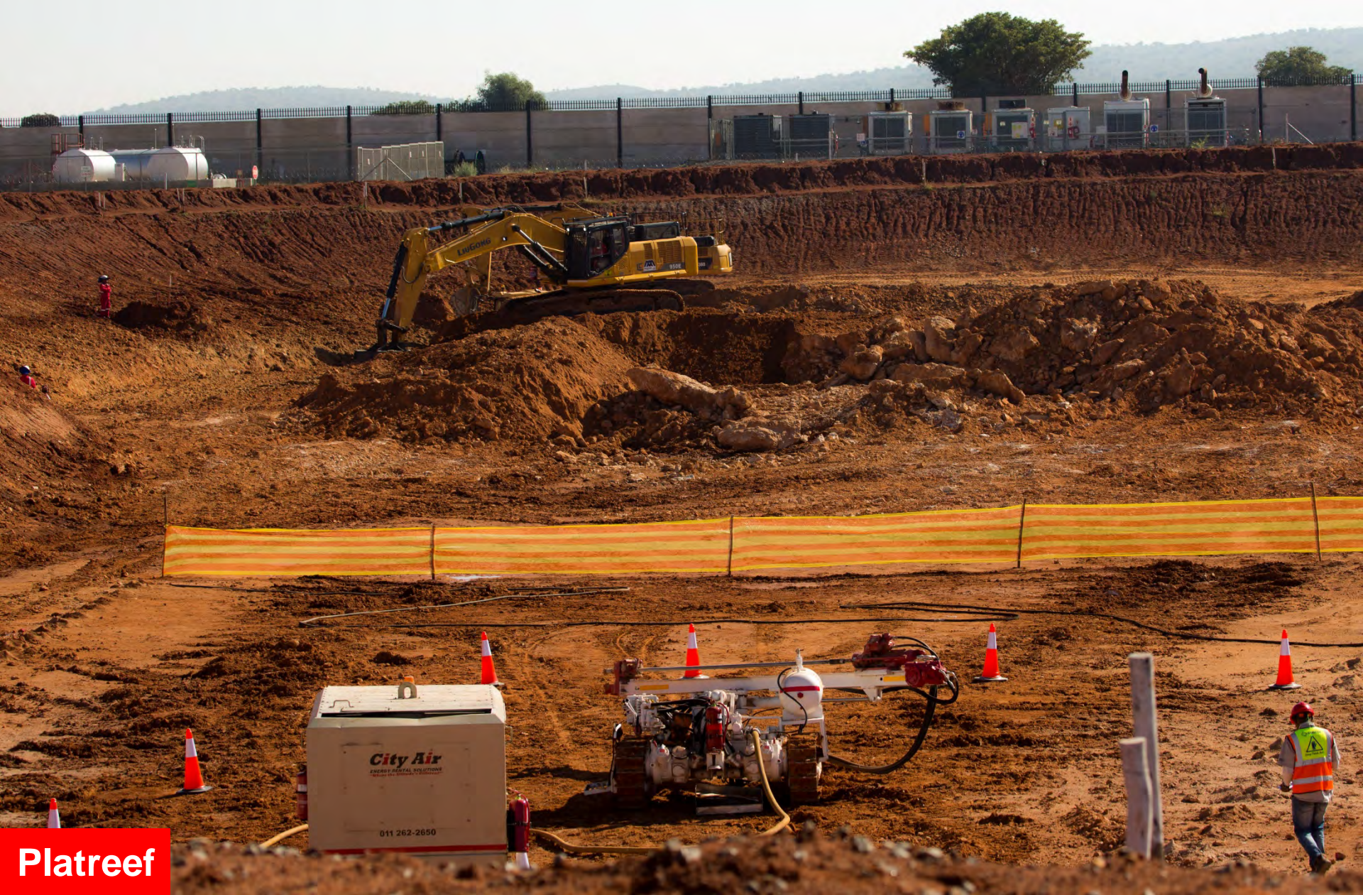
Preparation for blasting at the Shaft 2 box cut.
