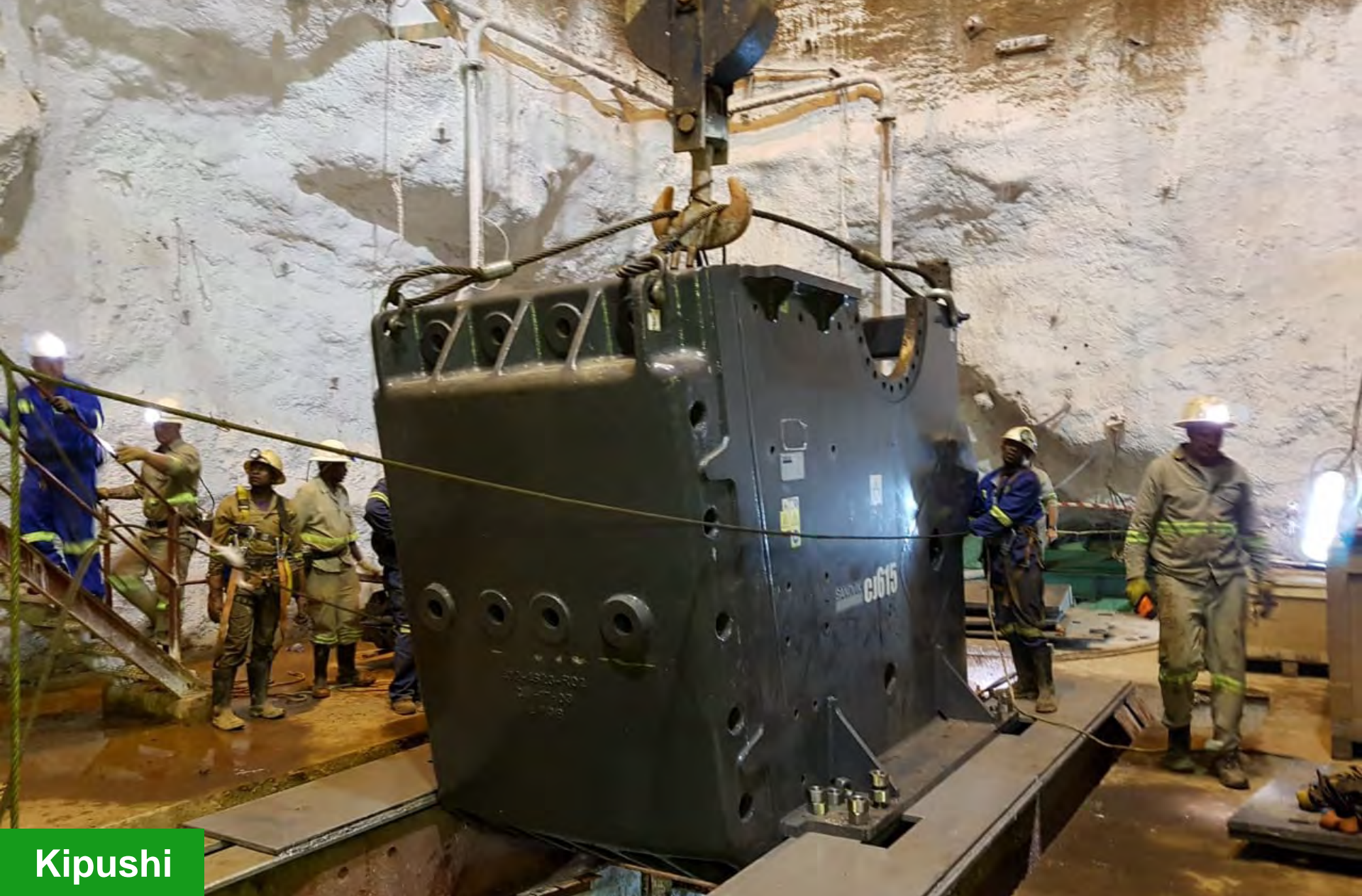
Main frame of the new underground rock crusher secured onto the base plate at the 1,150-metre level, ready for reassembly and commissioning.
