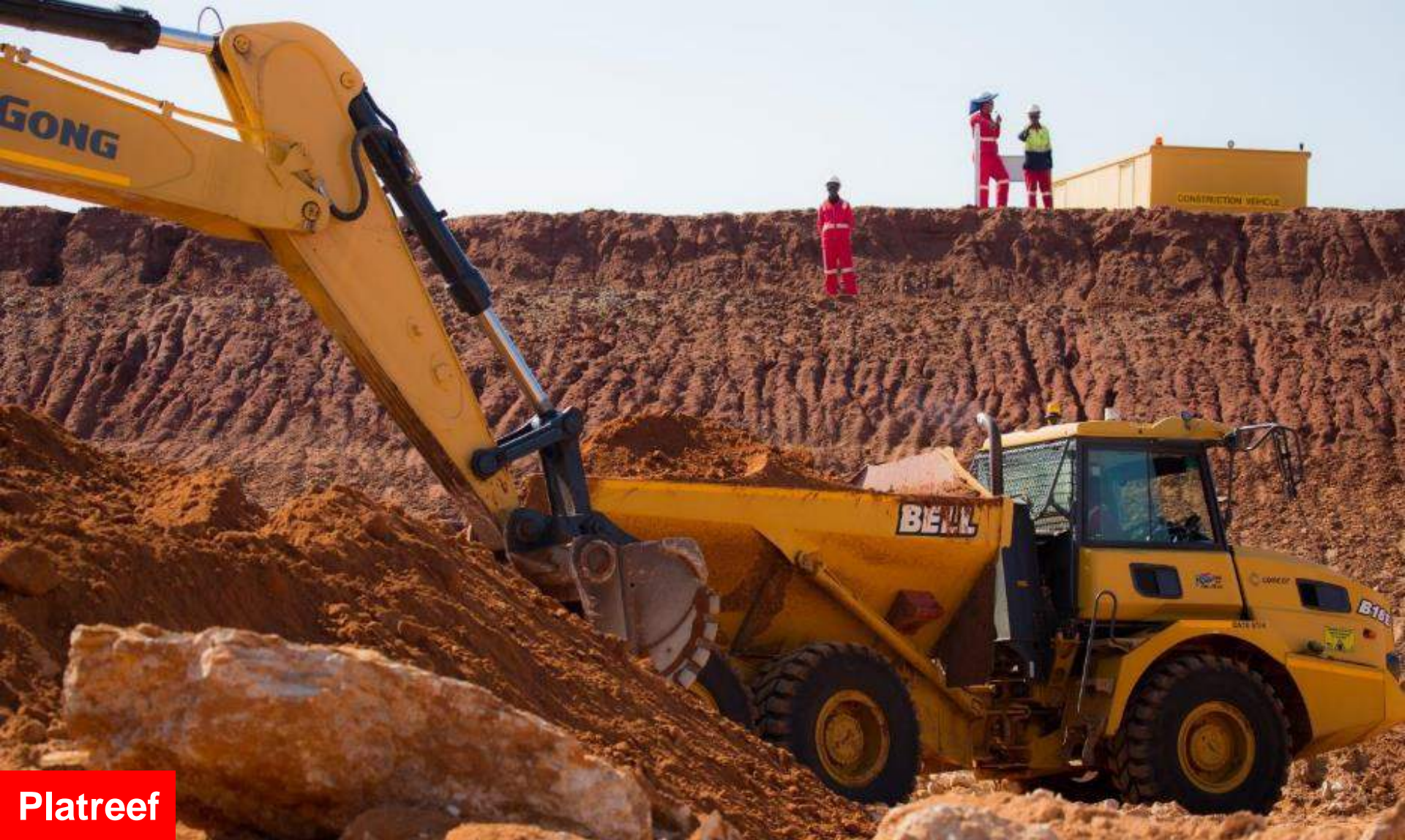
Removal of broken rock after a blast as part of the box-cut construction for Shaft 2.
