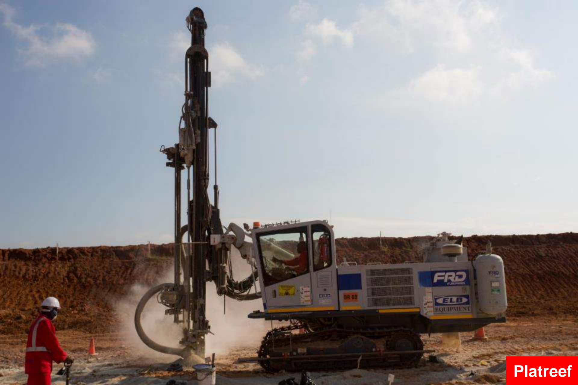
Drilling blast holes for the Shaft 2 box-cut construction.
