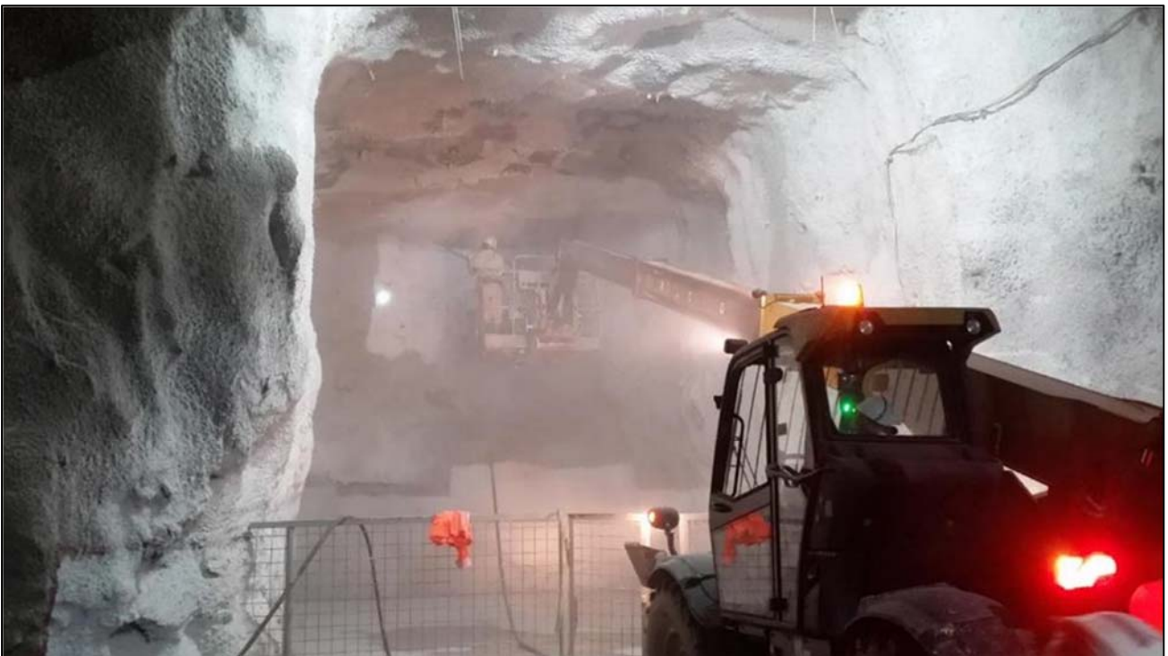
Figure 11: Workers scaling loose rock in one of Kakula's twin declines to prepare the working face for drilling. Both declines continue to make steady advancement toward the high-grade copper deposit.
