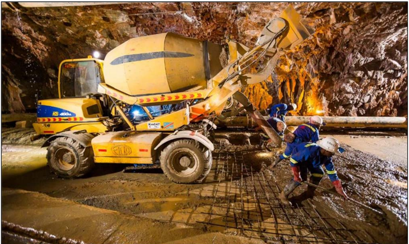
Figure 4: Pouring concrete for the new roadway on Kipushi's main haulage way at the 1,150-metre level.
