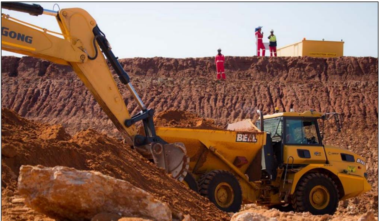
Figure 3: Removal of broken rock after a blast as part of the box-cut construction for Shaft 2.
