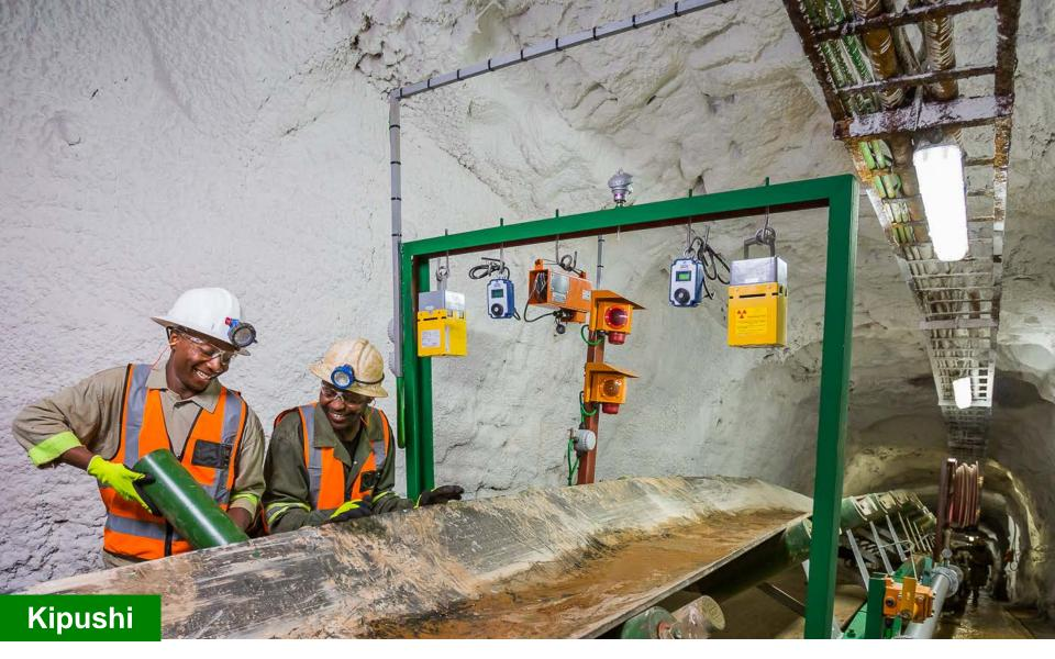
New rollers being installed on the ore conveyor on the Kipushi Mine's 1,150-metre-level as part of the infrastructure upgrading program.
