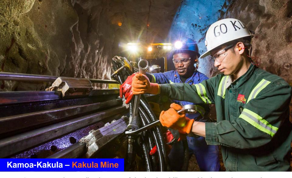
JMMC team members adjusting one of the jumbo drills used in the underground tunnelling operations that have advanced Kakula's twin declines approximately 400 metres toward the high-grade copper deposit.
