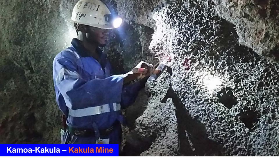
A member of the decline construction team testing the thickness of shotcrete applied to the walls of the conveyor decline at Kakula. Shotcrete is used to provide additional support in the underground excavations.
