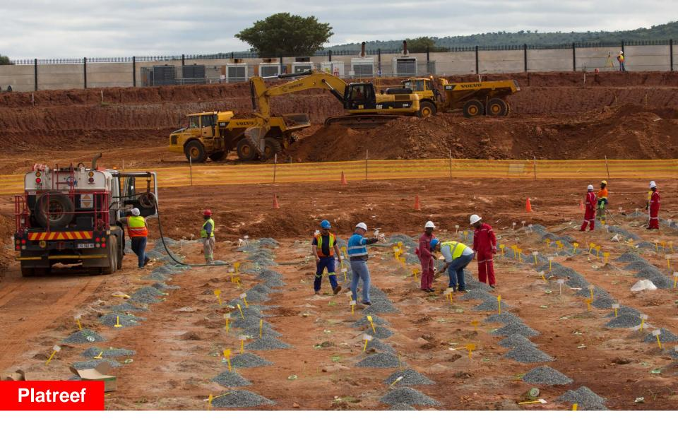
Loading explosives for the first blast for the Shaft 2 box cut development, which took place on April 12, 2018.
