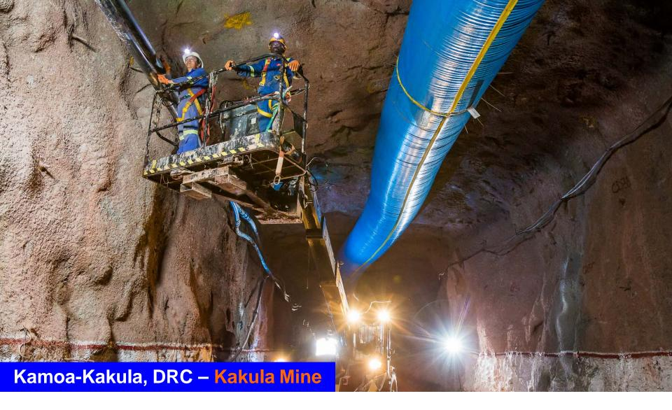
Workers with contractor JMMC installing water pipes and ventilation tubing in one of the twin declines at the Kakula Discovery.
