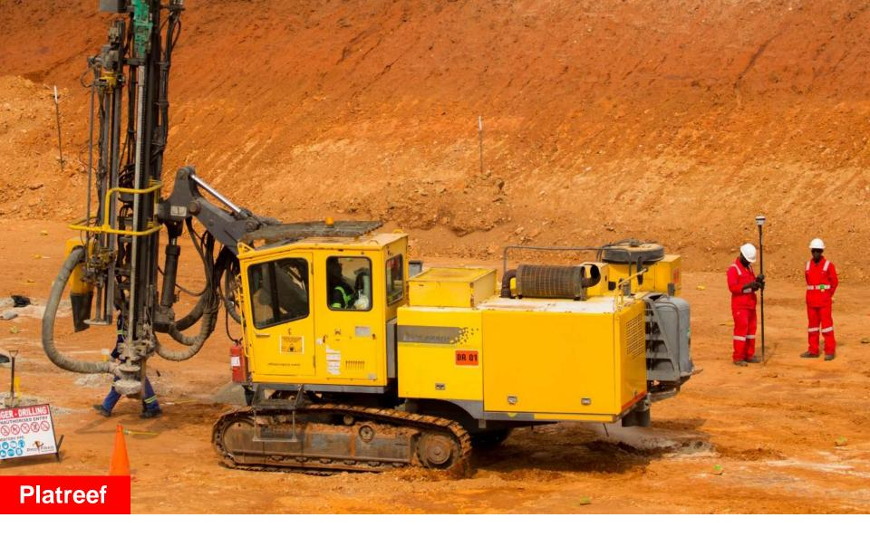
Drilling of blast holes as part of early-works construction for Shaft 2 at the Platreef Mine in South Africa.
