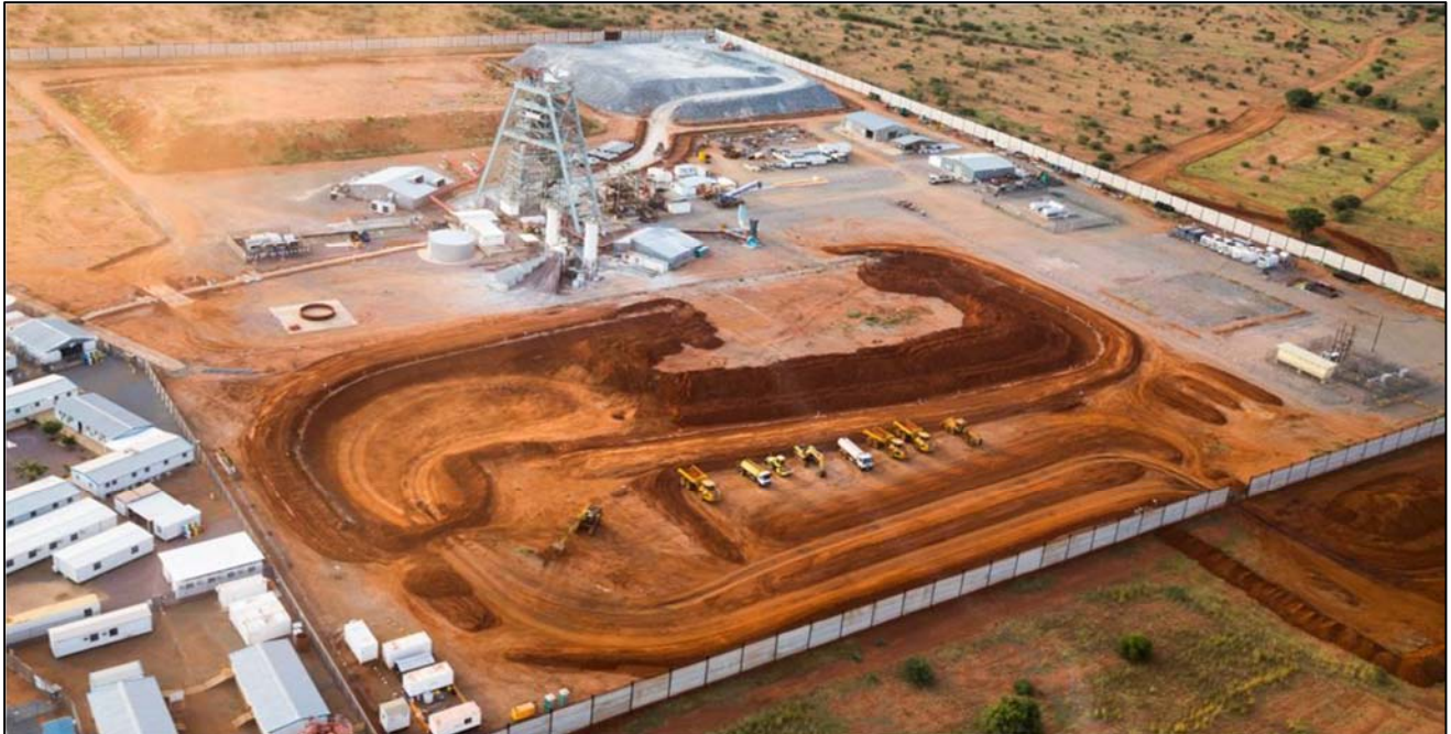
Figure 2: Excavation of a surface box cut now underway as part of early-works construction for Shaft 2 at the Platreef Mine in South Africa.
