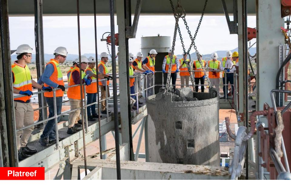
Site visitors at the top of Shaft 1 viewing excavated rock from shaft-sinking operations being hoisted in a kibble bucket.
