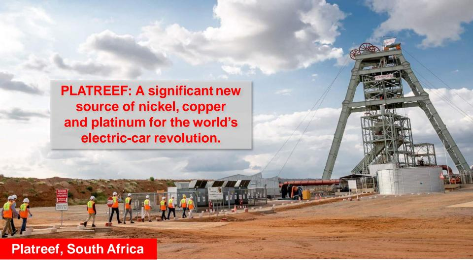
Investors arriving at Shaft 1 on a recent visit to the Platreef Project. The shaft, 7.25 metres in diameter, is expected to reach the Flatreef mineralization at a depth of approximately 780 metres in the third quarter of this year.
