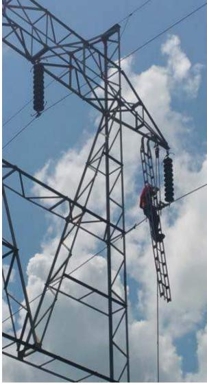
Installation of lightning-protection wire completed on a new 6.6-kilovolt overhead power line by contractor, PANACO. The new lines deliver power to pump stations that supply drinking water to residents of the town of Kipushi as part of Ivanhoe's community-support initiatives.
