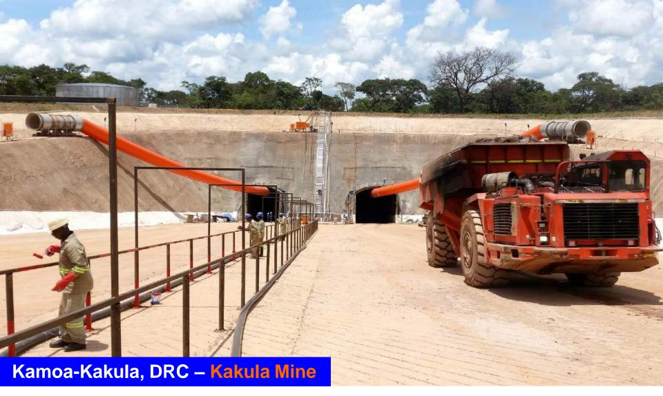
Excavated rock being hauled out of the services decline at the planned Kakula Mine. Underground development work on the twin declines is progressing ahead of plan. Both declines have been advanced more than 300 metres toward the high-grade copper deposit.
