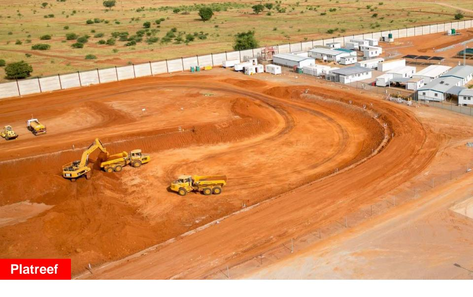
View from the top of Shaft 1 of the excavation site for the 29-metre-deep box cut for Platreef's Shaft 2.
