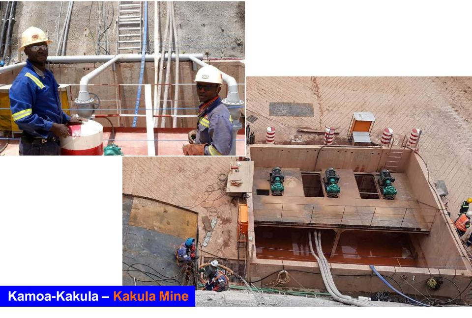
Water sump being completed at the bottom of the Kakula box cut by construction team members.
