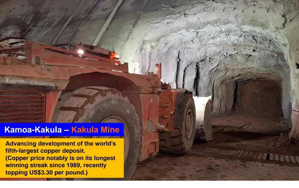
A scoop-loader removing excavated rock from the services decline that's continuing to advance toward the high-grade copper resources for the planned Kakula Mine.
