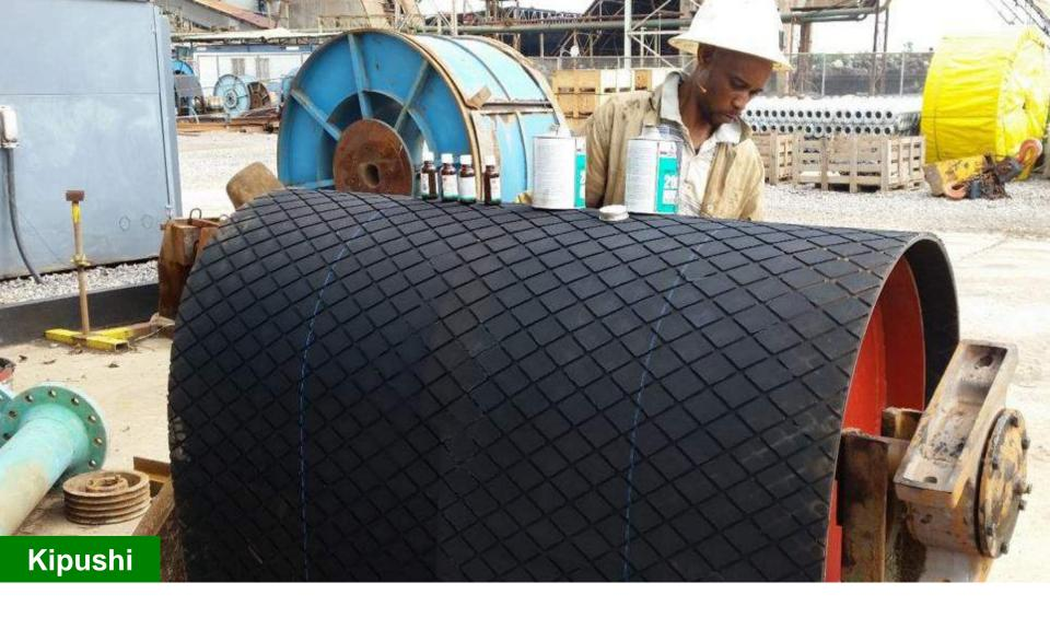
Rubber lagging being wrapped and glued on a pulley that will help to guide and drive the belt on the ore conveyor at Shaft 5.
