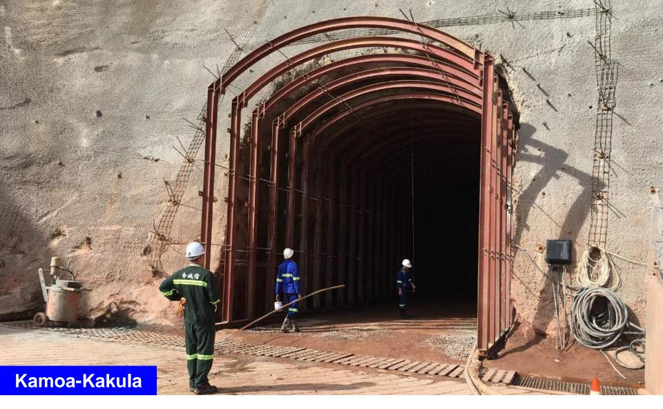
Installation of steel sets for roof and wall support in the services decline for the Kakula Mine. The services decline is one of two adjacent ramps that will provide underground access to the high-grade deposit.
