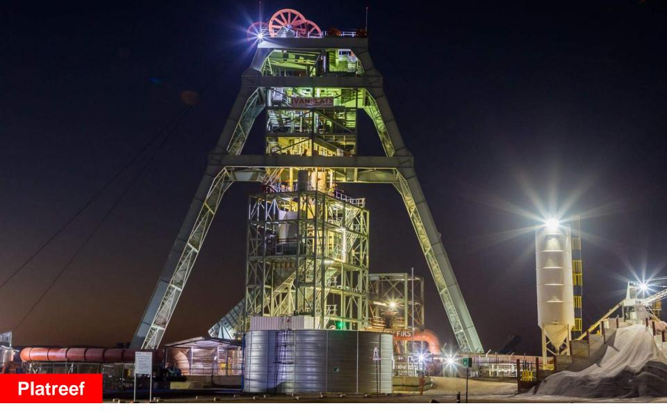
The 7.25-metre-diameter Shaft 1, expected to reach the Flatreef mineralization at a depth of approximately 783 metres in the third quarter of this year, will be used for initial access to the Flatreef Deposit and early underground development.
