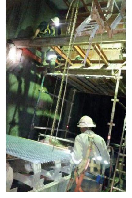
Maintenance and engineering team members installing a new platform at the mine's T2 loading area – part of the underground conveyor system.
