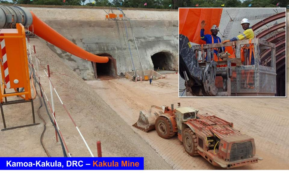
Ventilation system being installed in the mine-access declines at the Kakula box cut by members of the Kakula Mine development team.
