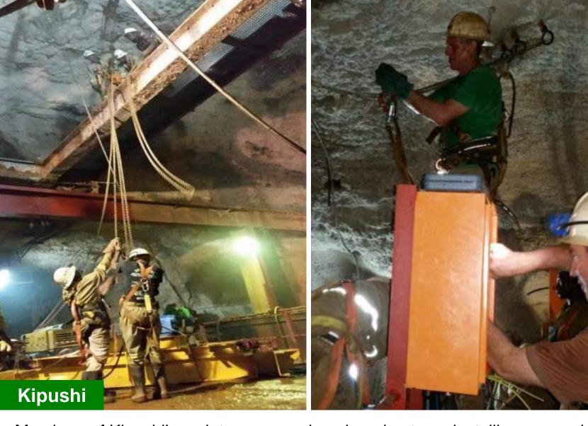
Members of Kipushi's maintenance and engineering team installing an overhead crane that was recovered from the earlier plant.
