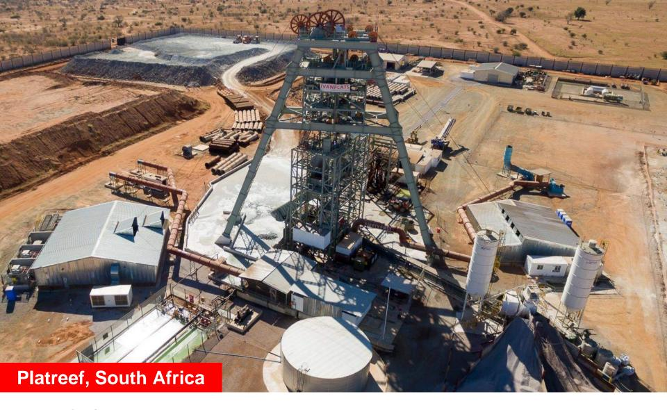
Platreef's Shaft 1, now more than 580 metres below surface, will provide early development access into the Flatreef Deposit and will be utilized to advance production of platinum-group elements, nickel, copper and gold.
