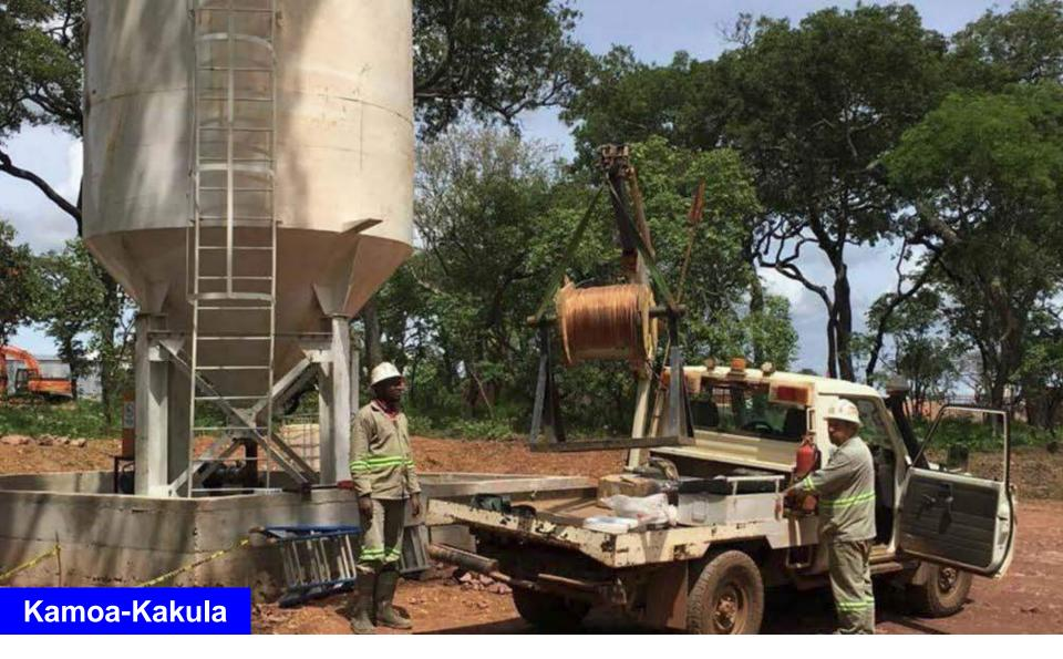
Installation of electrical wiring on an emulsion plant that will provide explosives for the decline development underway at the Kakula Mine.
