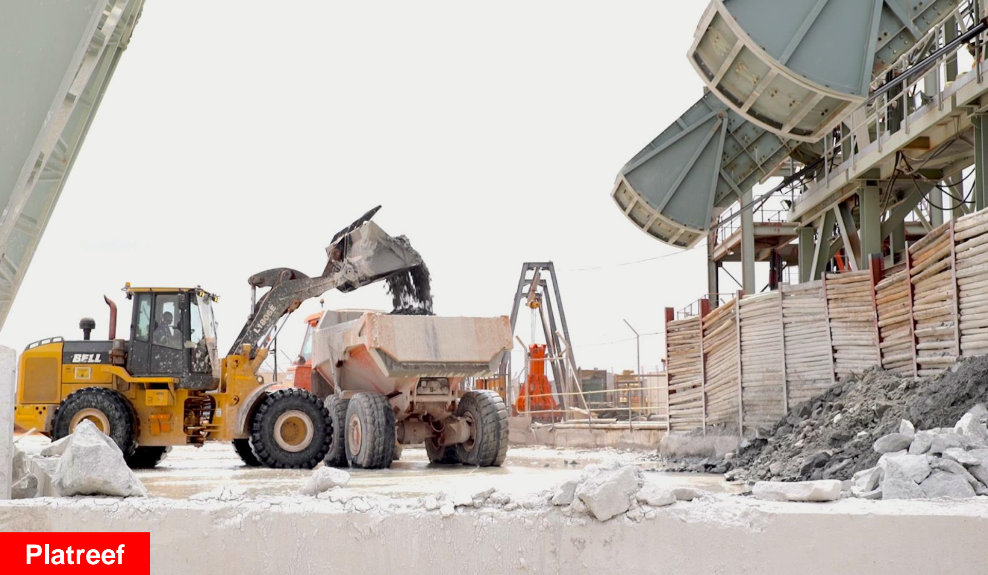
Muck-clearing operations during a cleaning cycle in ongoing sinking work at Shaft 1.
