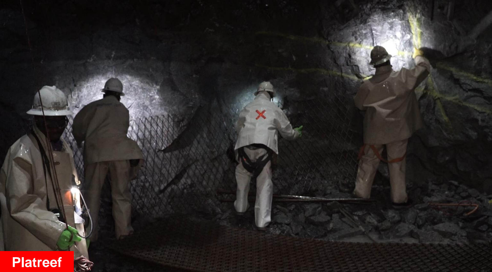
Workers installing steel strapping and wire mesh to exposed walls in Shaft 1 as a safety measure to prevent loose rocks from falling during sinking activities.
