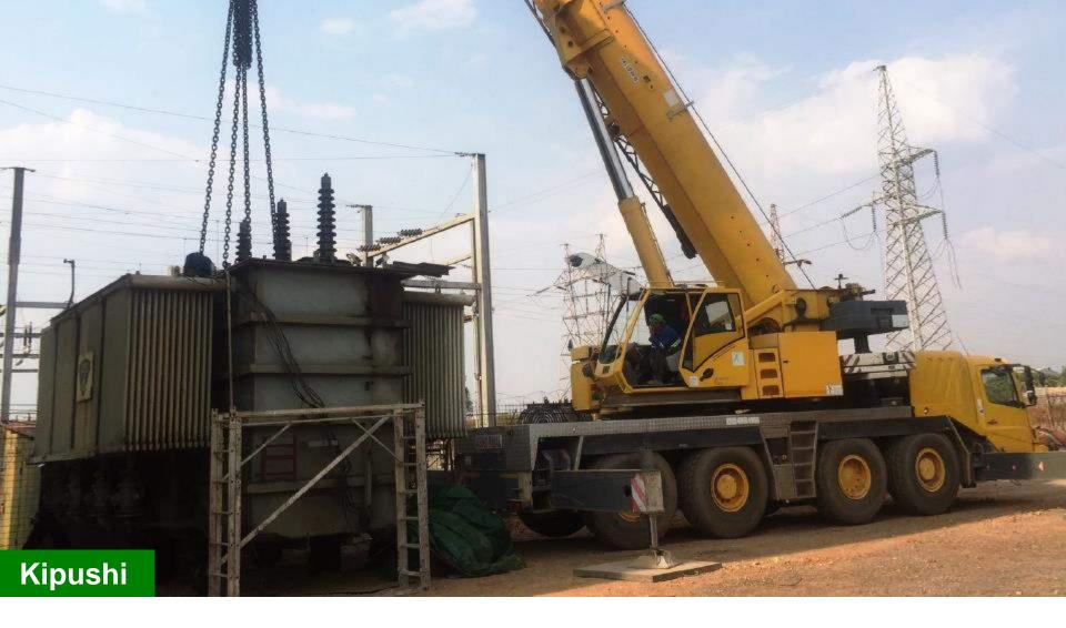
A 45-kilovolt transformer at Kipushi's electrical substation undergoing upgrading work.
