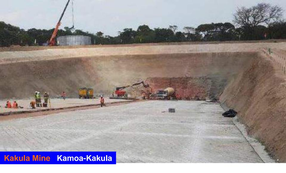
Concrete ramp in the Kakula box cut will be used to transport excavated rock to surface stockpiles during the development of the twin declines.
