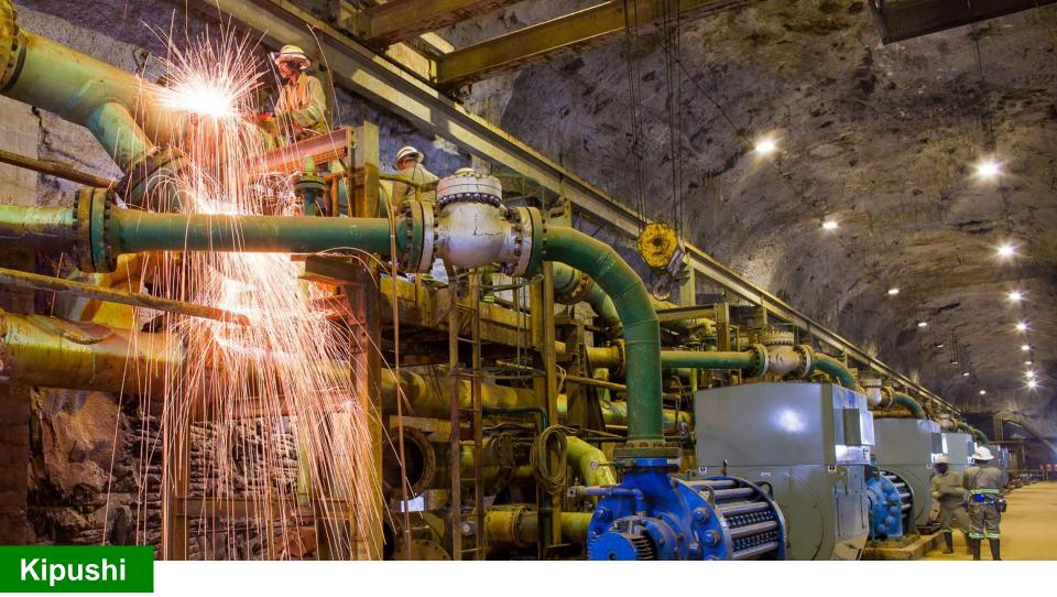
Welding at the Kipushi Mine's Shaft 5 pumping station in preparation for a resumption of production.
