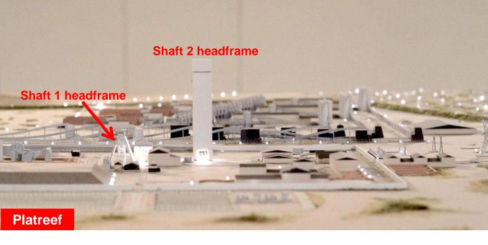
A model of the planned Platreef Mine showing headframes for shafts 1 and 2, and processing infrastructure.
