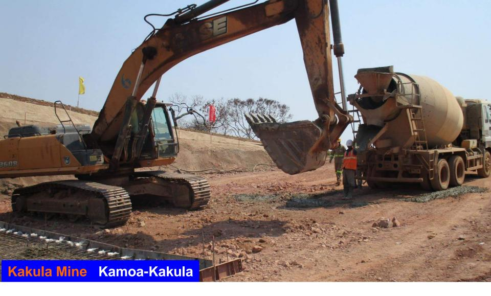
Preparing to pour concrete during roadway construction at the Kakula box cut.
