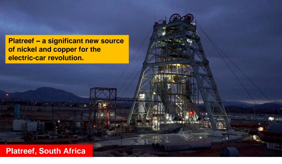
Shaft 1 has reached a depth of more than 500 metres below surface as mine development advances. The 7.25-metre-diameter Shaft 1 is expected to reach the Flatreef mineralization at a depth of approximately 783 metres in the third quarter of next year.
