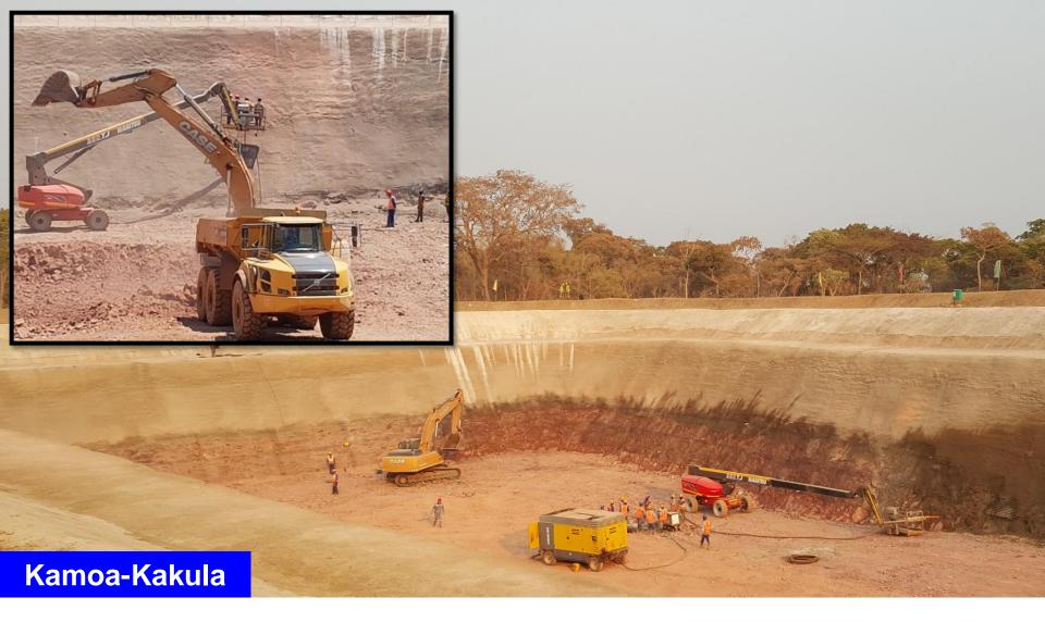
Heavy equipment removing excavated rock from the planned 18-metre-deep Kakula box cut. Excavation, support and civil works are on track to be completed by the end of October 2017.
