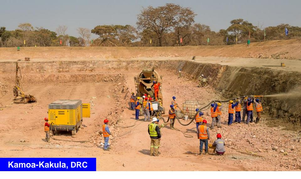
Workers spraying shotcrete (a wet concrete mixture) onto wire mesh to support sidewalls during excavation of the Kakula box cut.
