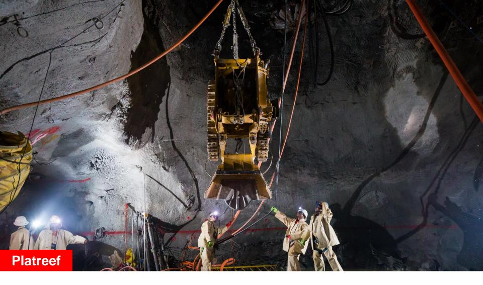
Excavation equipment lowered into Shaft 1 to remove rock during development of the 450-metre-level station.
