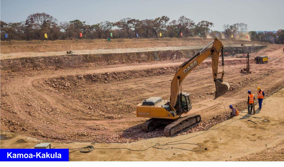
Removal of excavated rock from the site of the box cut for the planned Kakula Mine – the second mine development underway at the Kamoa-Kakula Project – and drilling in preparation for the second blast to take the box cut to a depth of 18 metres below surface.
