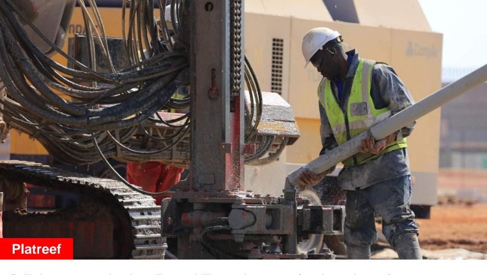
Drill-rig crew member installing a drilling rod as part of early-works surface construction at Shaft 2. Early works will consist of a box cut to a depth of approximately 29 metres below surface and construction of the concrete hitch (foundation) for the 103-metre-tall concrete headgear (headframe) that will house the shaft's permanent hoisting facilities and support the shaft collar.
