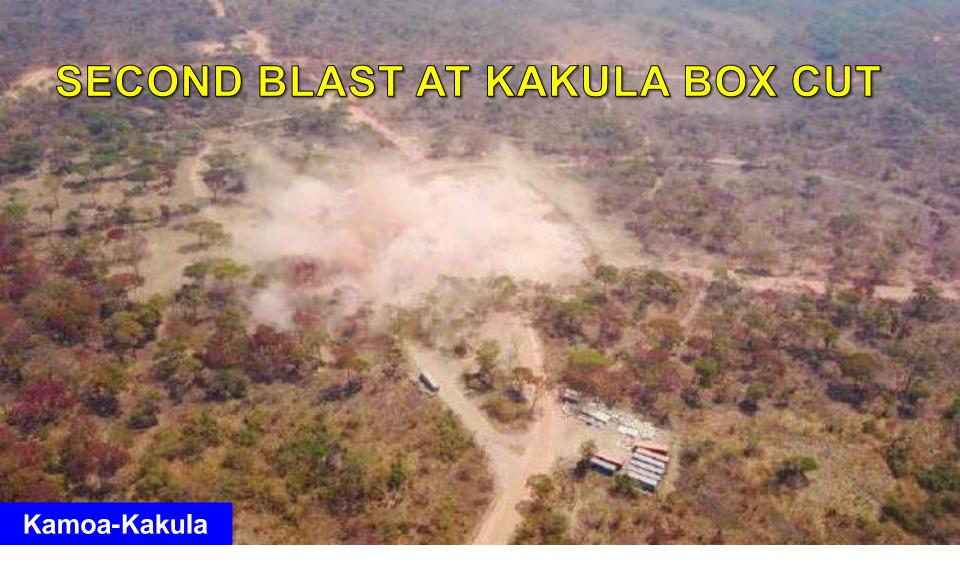
The second blast at the box cut for the Kakula Mine was detonated on August 16. Construction of twin tunnels in the box cut is expected to begin this November. The 1,500-metre-long tunnels will reach the ultra-high-grade Kakula Discovery 250 metres below surface.
