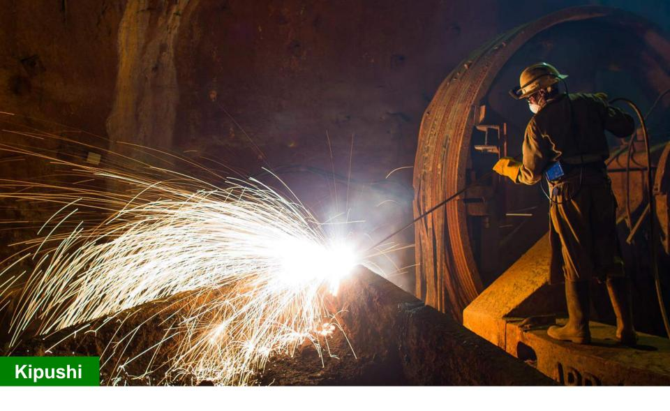
Welding at the underground primary crusher as part of the upgrading and modernizing of the Kipushi Mine in preparation for the restart of commercial production.
