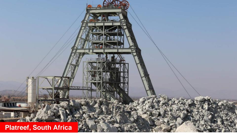
Headgear and infrastructure at Platreef Project's Shaft 1. Excavated rock in foreground is from shaft-sinking and underground development. Shaft-sinking is expected to resume in mid-September, following completion of the initial shaft station at the 450-metre level.
