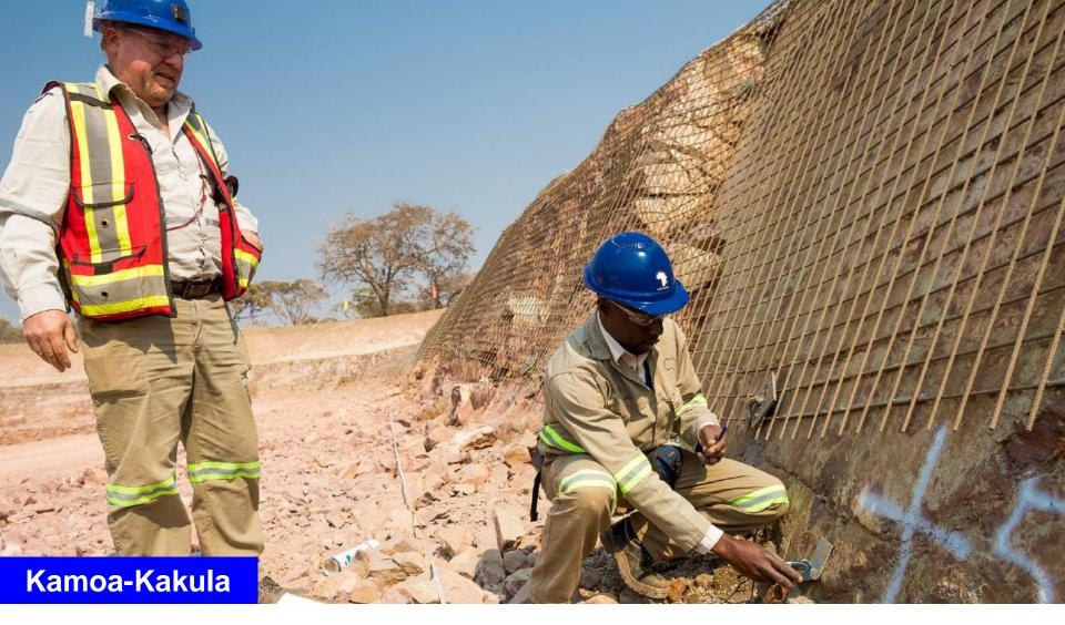
Measuring the slope angle of the side wall at the Kakula box cut.
