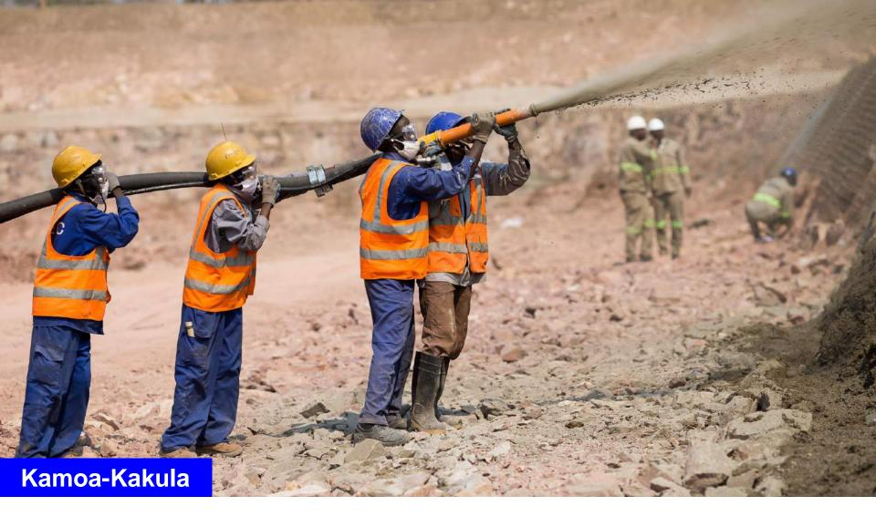
Workers spraying shotcrete (a wet concrete mixture) onto wire mesh along the sidewalls of the Kakula box cut to help stabilize and provide support for the excavated box-cut walls.
