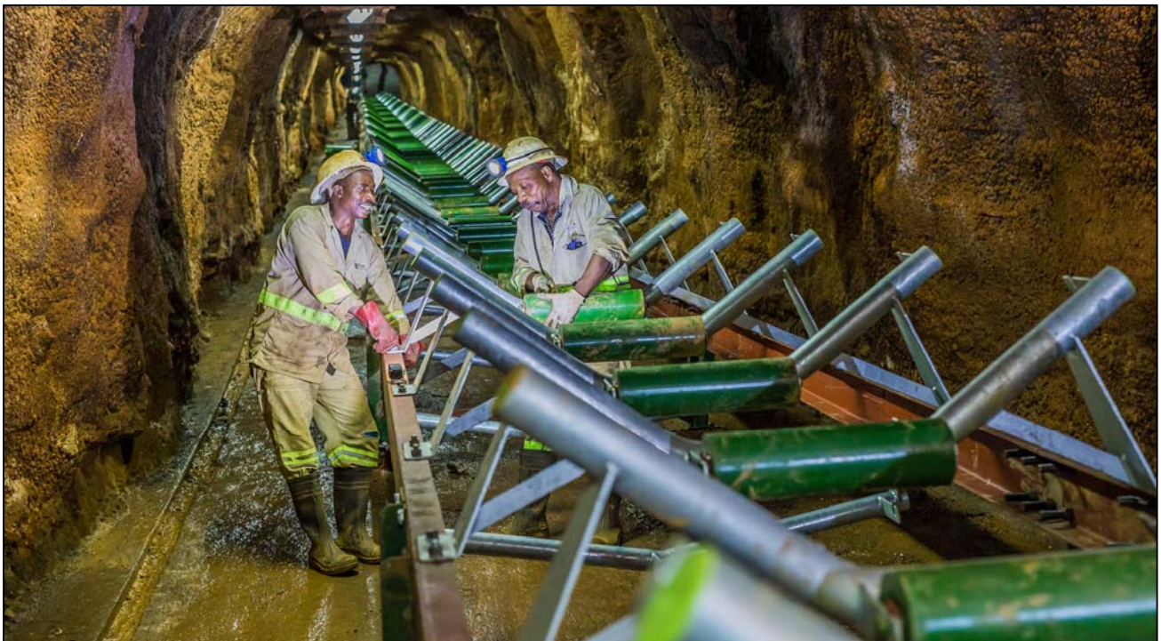
Figures 6 and 7: Installation of conveyor belt rollers in Shaft 5 ore load-out system.
