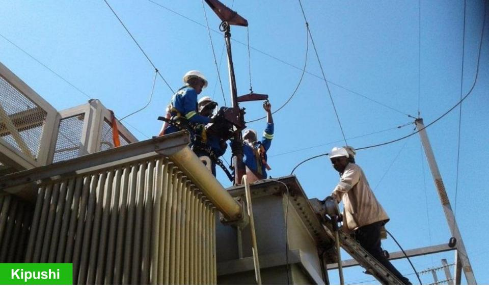
Upgrading a 45-megavolt-ampere transformer at the Kipushi Mine.
