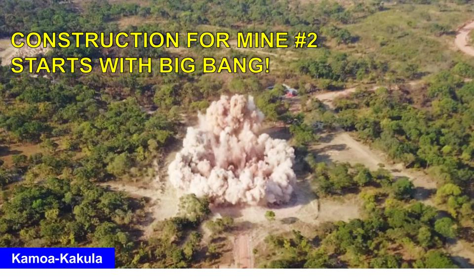
The first blast marking the start of construction at the Kakula box cut was triggered on June 28. The box cut will provide entry to twin tunnels, each approximately 1,500 metres long, planned to reach the ultra-high-grade Kakula Discovery around 250 metres below surface.
