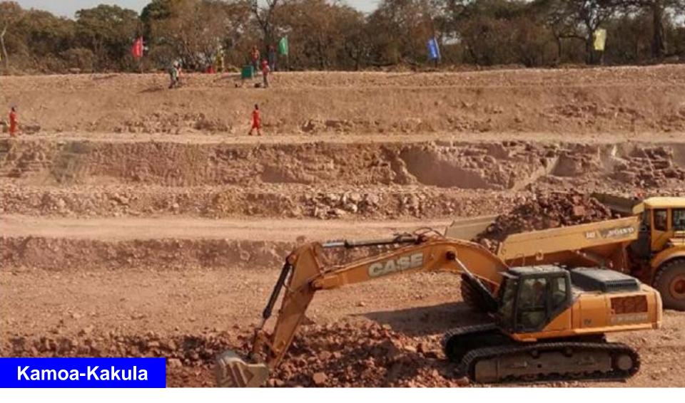
Heavy equipment removing broken rock from the Kakula box cut, which will be 18 metres deep and is expected to be completed in October 2017.
