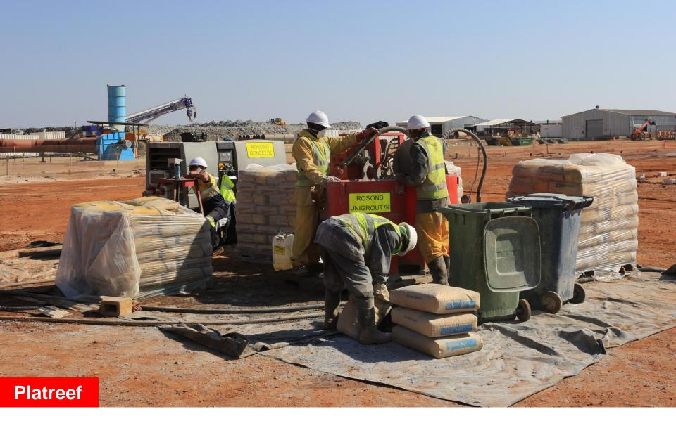
Cement mix for grouting operations underway at Platreef's Shaft 2.
