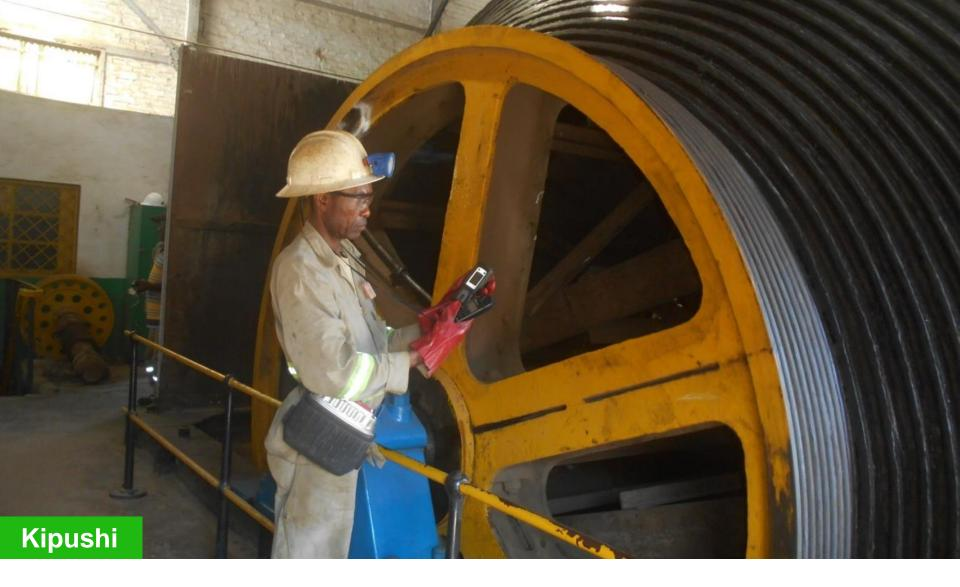
Routine testing of Kipushi's Shaft 5 hoisting winder.
