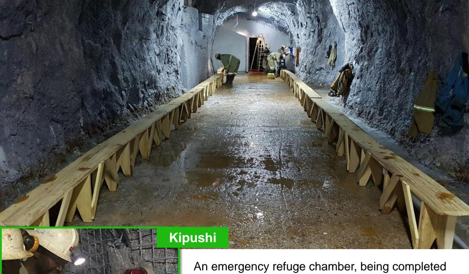
An emergency refuge chamber, being completed and equipped 1,132 metres below surface, is a key worker-safety facility added as part of the upgrading of the Kipushi Mine.
