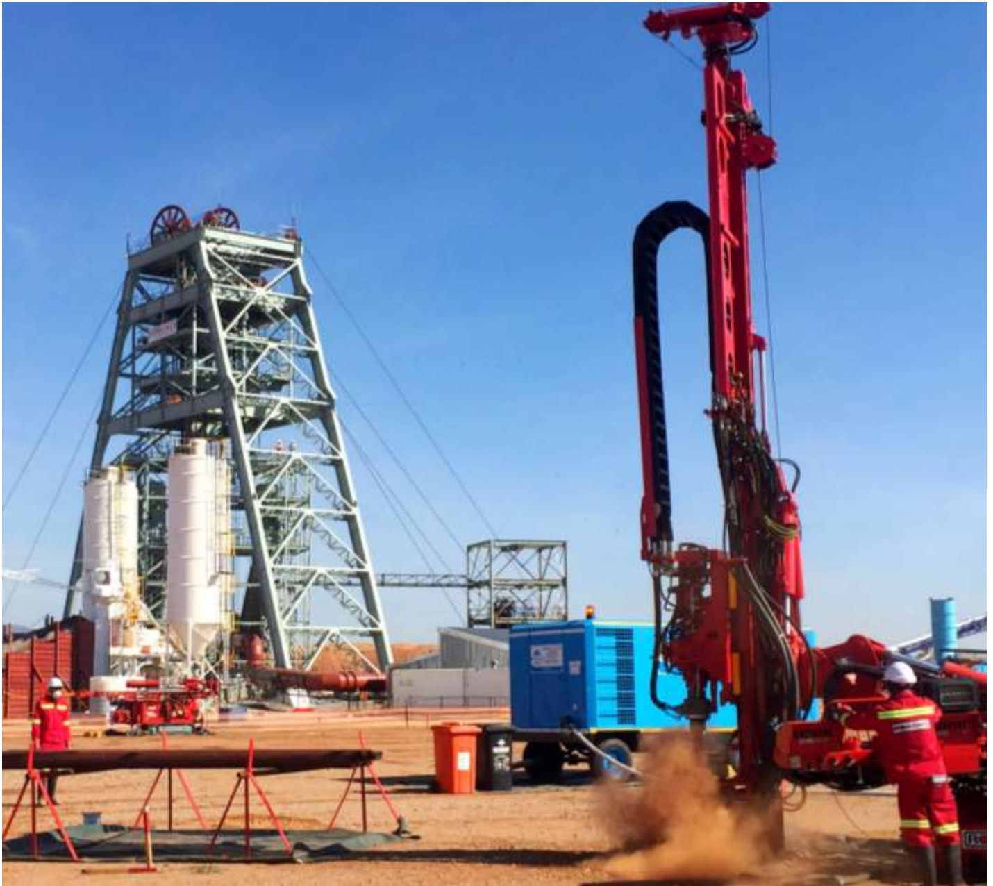
Photo 5: Shaft 2 early works underway.
