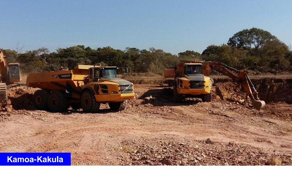
Work is underway for the construction of a box cut at the Kakula Discovery to accommodate twin decline ramps that will provide underground access to the Kakula ultra high-grade deposit.
