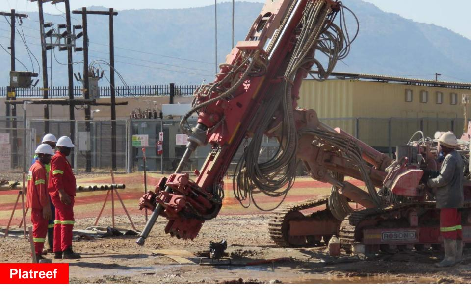
Operation of a Rosond drill rig as part of early-works construction at Platreef's Shaft 2.
