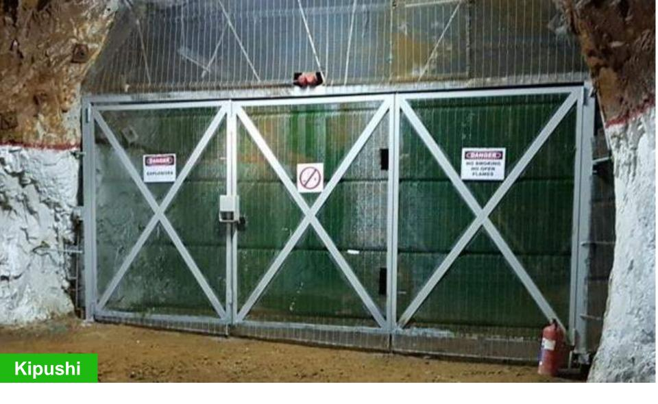
A new explosives storage area constructed at the 1,132-metre level as part of Kipushi's infrastructure upgrading program.
