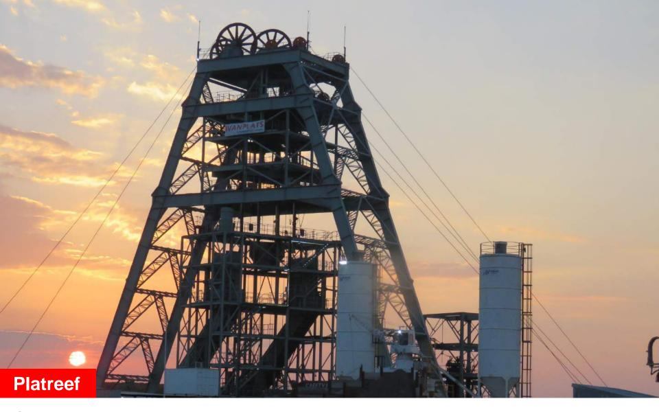
Shaft 1, now sinking at a rate of approximately 45 to 50 metres per month, will provide development access into the Flatreef Deposit while Shaft 2 is being developed.
