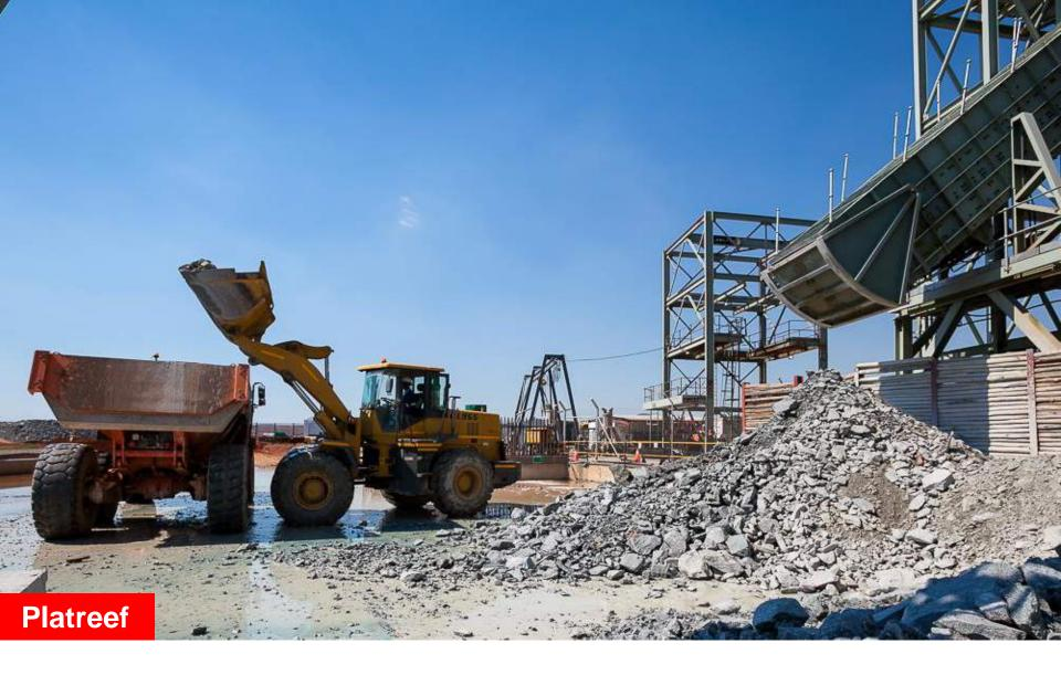
Removal of excavated rock during shaft-sinking operations.
