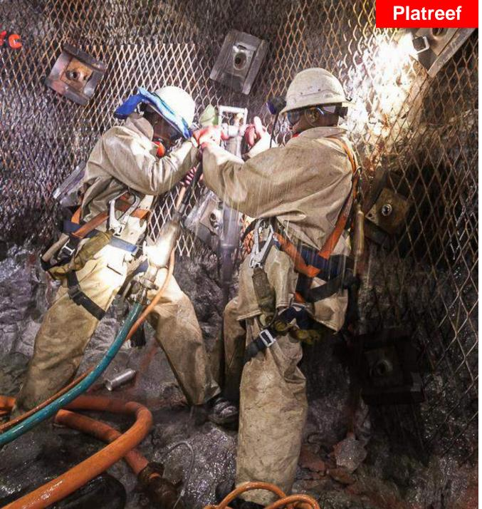
Platreef sinking team members drilling a hole during the ongoing shaft sinking of Shaft 1.
