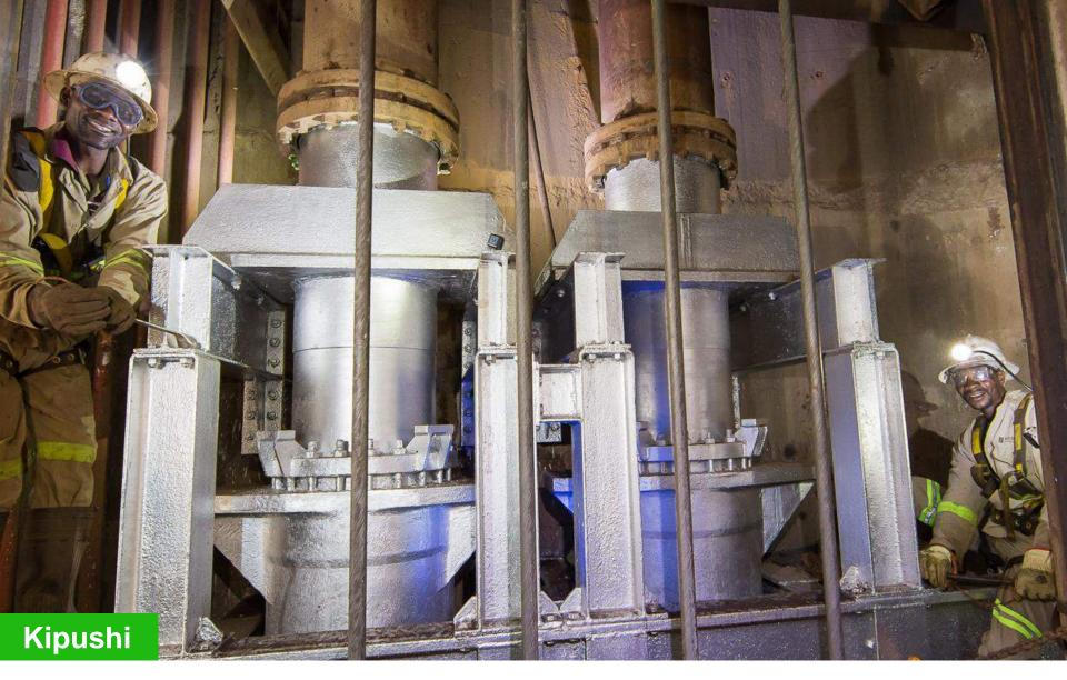
Upgraded supports for Shaft 5 pump columns at the 1,200-metre-level pump station.
