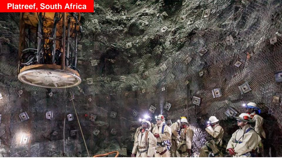
Members of the Platreef sinking team in Shaft 1, which now is at a depth of approximately 300 metres below surface. Sinking is continuing to a planned final depth of 980 metres. Shaft 1 will provide access into the Flatreef Deposit during the development of Shaft 2, the project's main production shaft.
