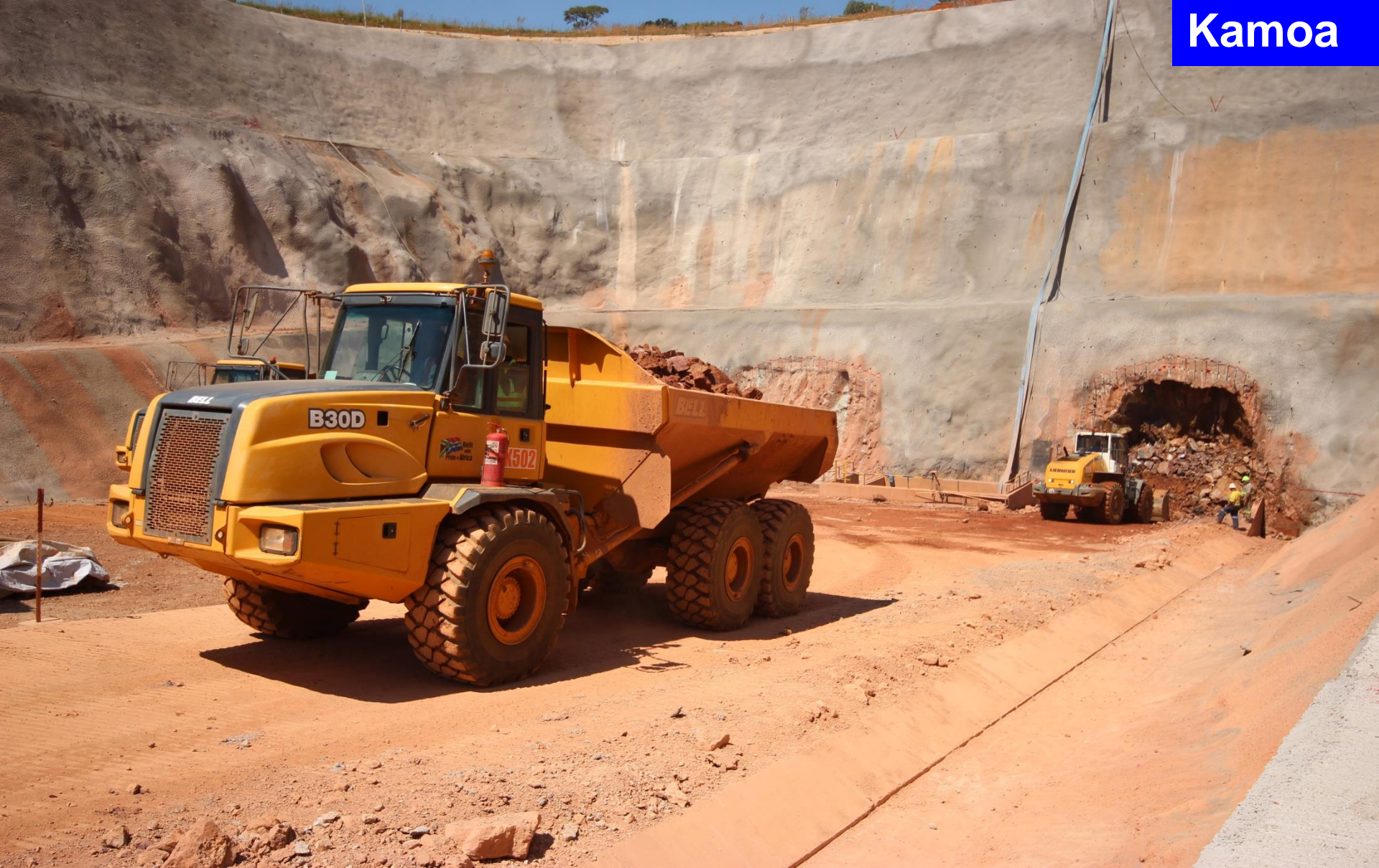
Broken rock being removed after the first blast.
