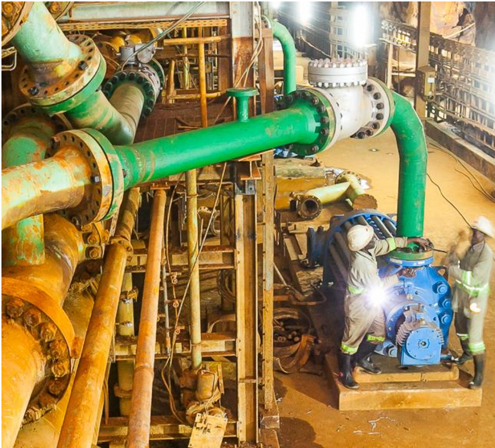
Workers installing a new Grifo pump at the 1,200-metre pump station.
