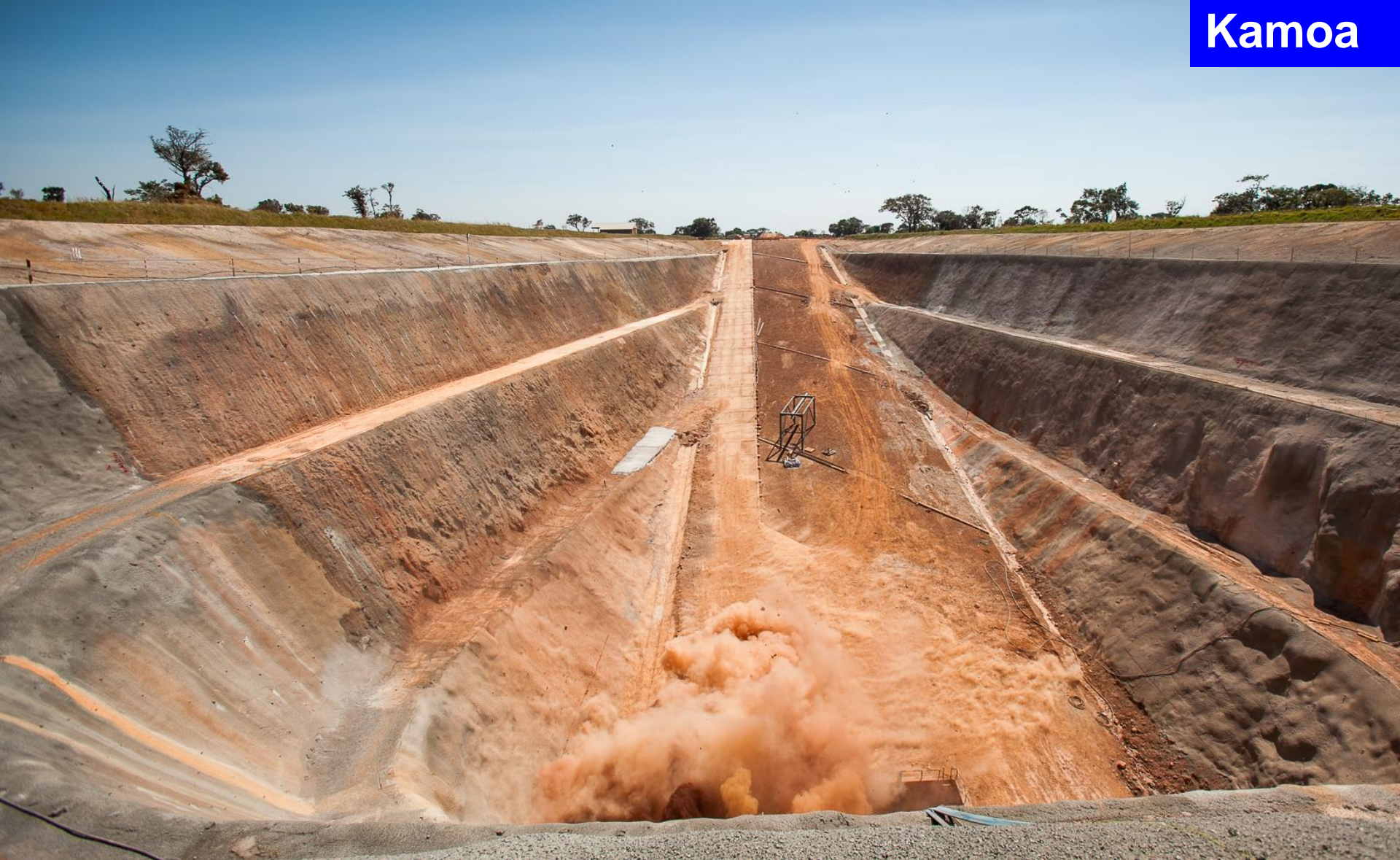
First excavation blast for the twin declines at the bottom of the box cut.
