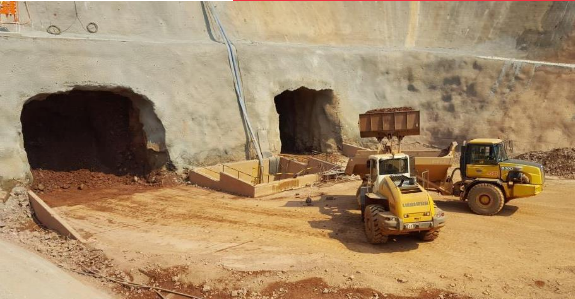
Broken rock being removed from the twin declines at the Kamoa box cut that will provide access to the planned underground mine at Kansoko Sud.
