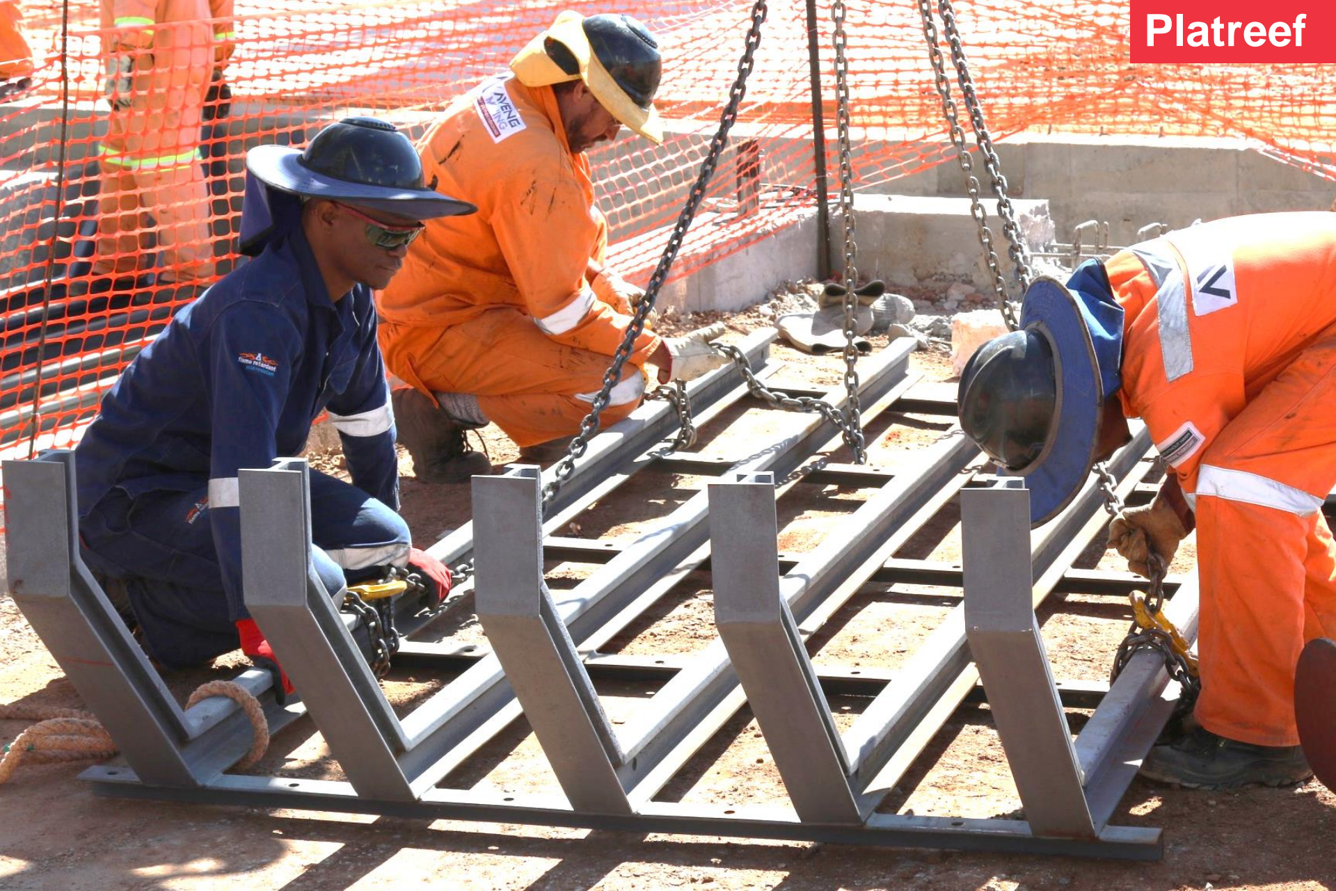
Guide beams for the jumbo drill rig at Shaft 1.
