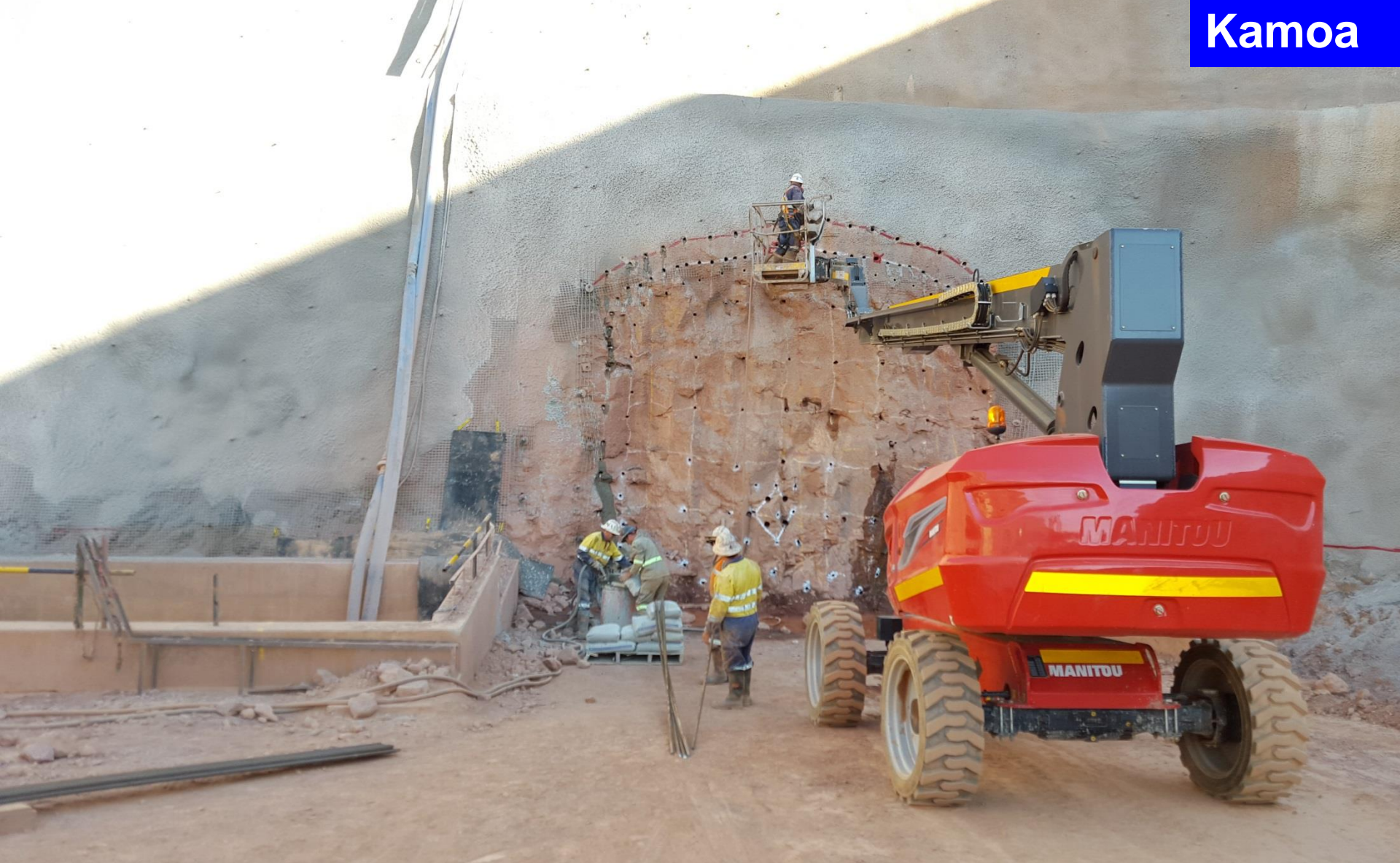
Preparing for the first blast at the Kamoa box-cut declines.
