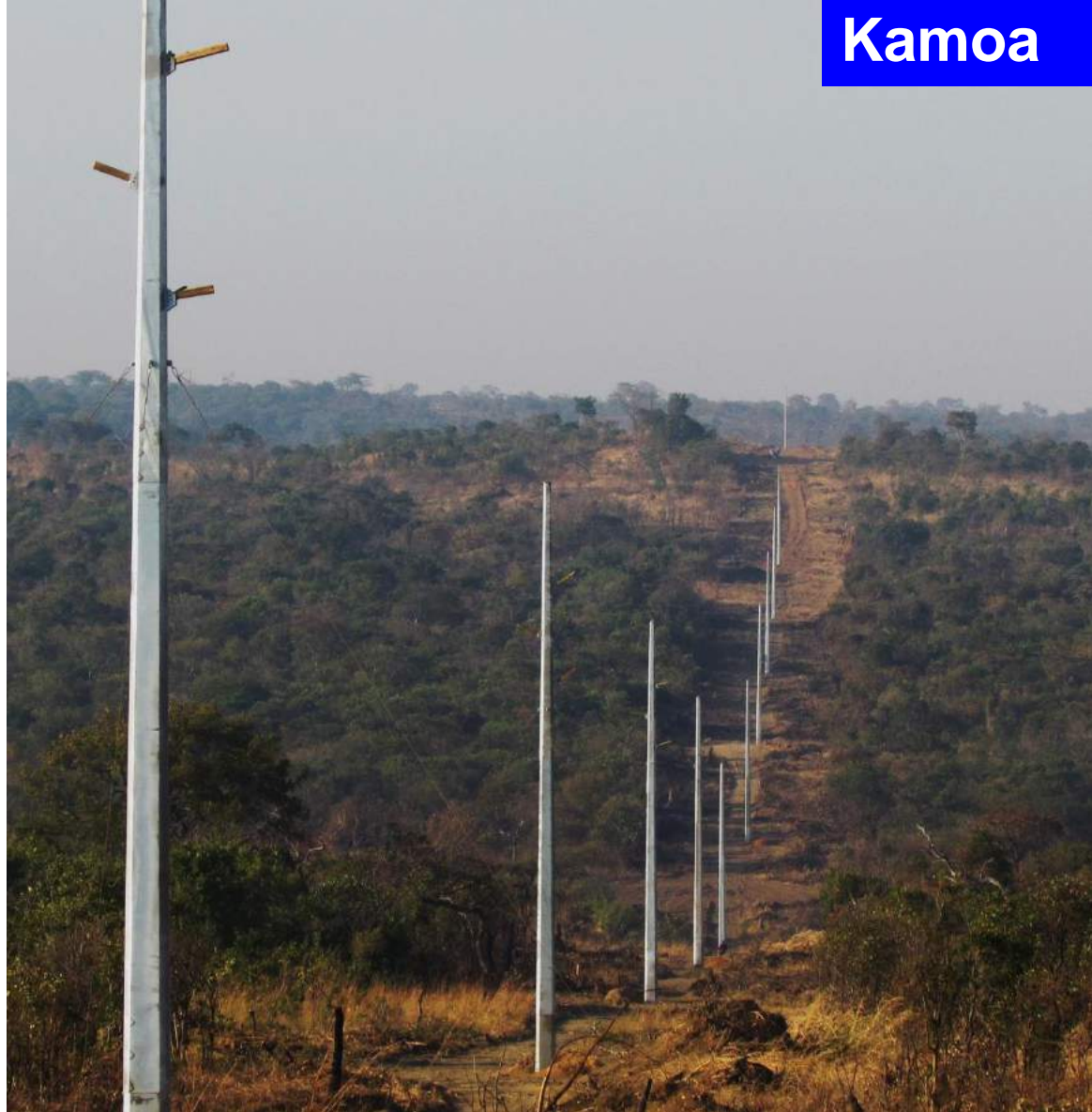
Installation of a 120kV power line at the Kamoa Project.
