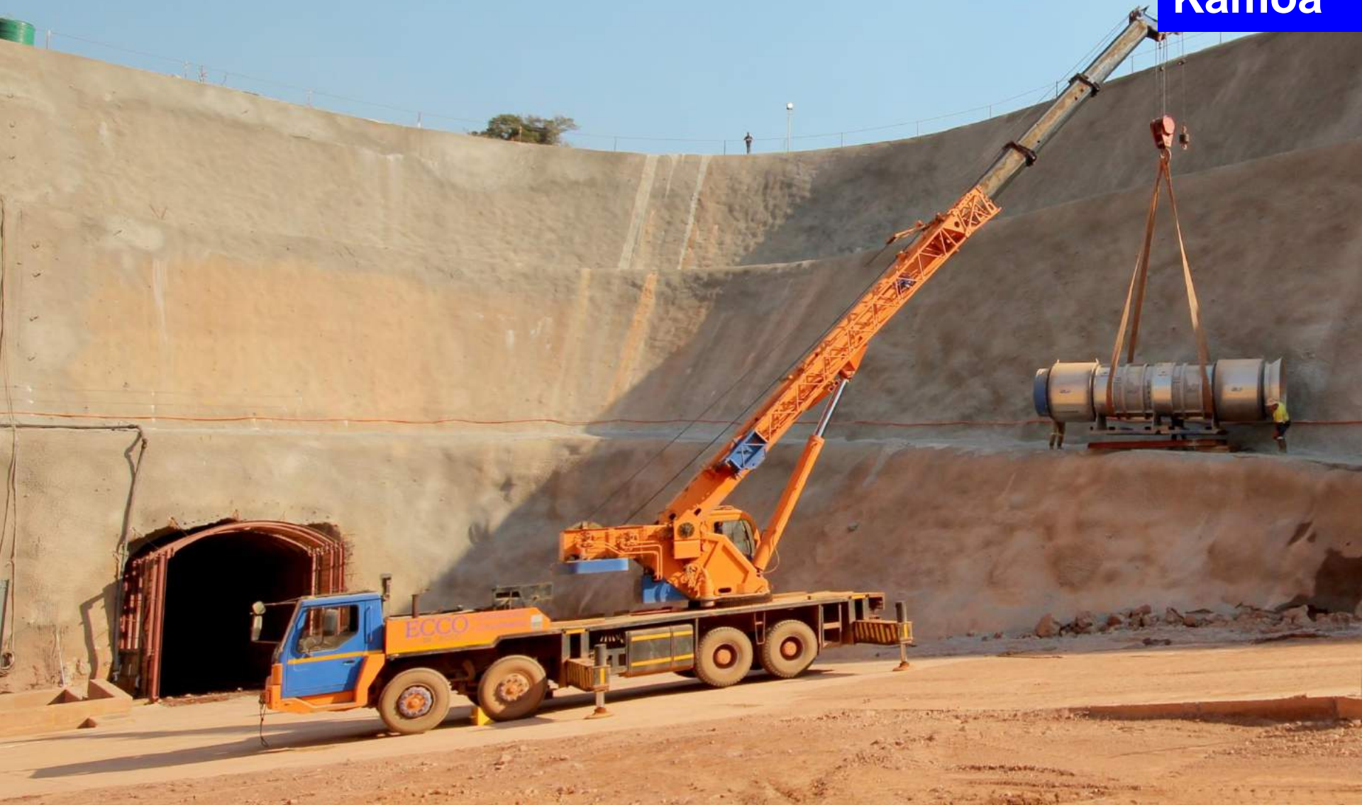
Unloading a ventilation fan to be installed at the Kamoa box cut.
