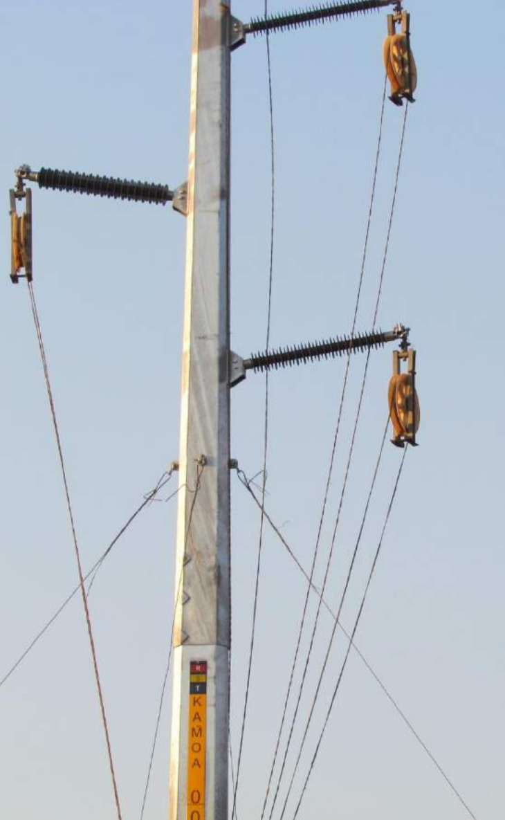
Installation of a 120kV power line at the Kamoa Project.
