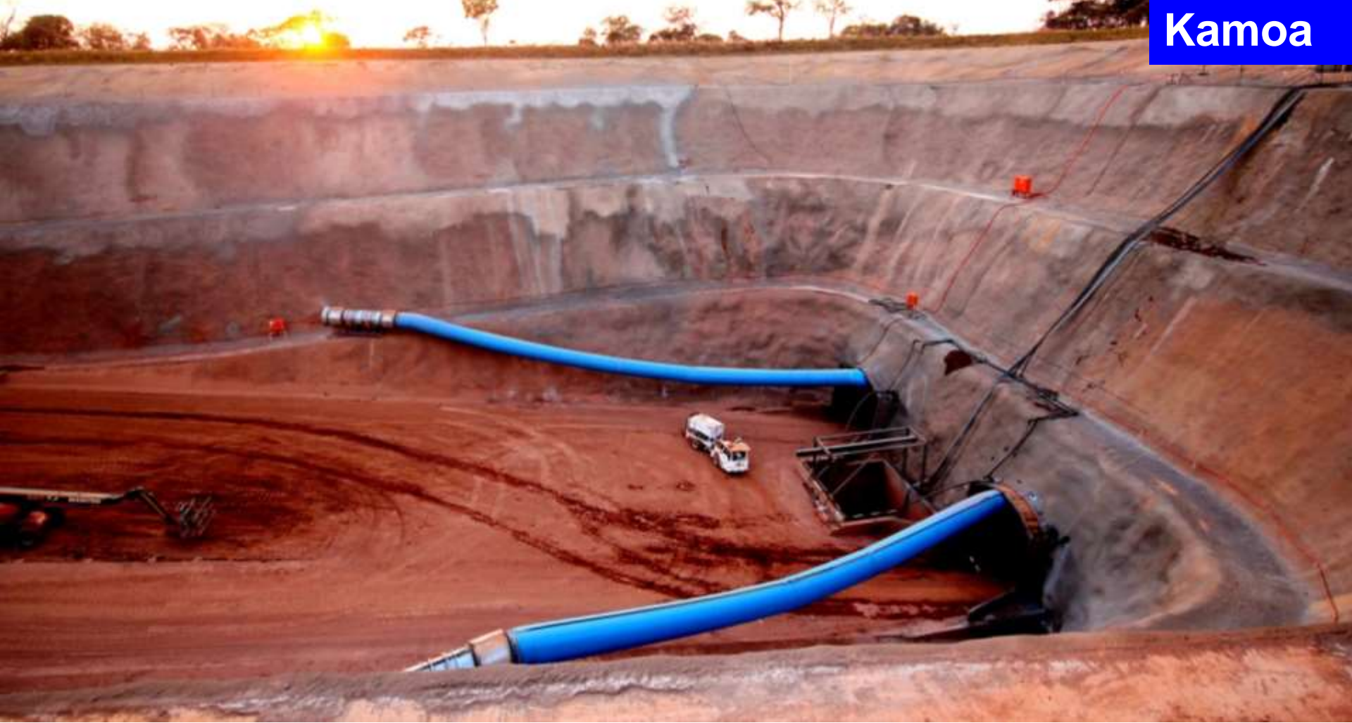
Ventilation system for the mine portals at the Kamoa box cut.
