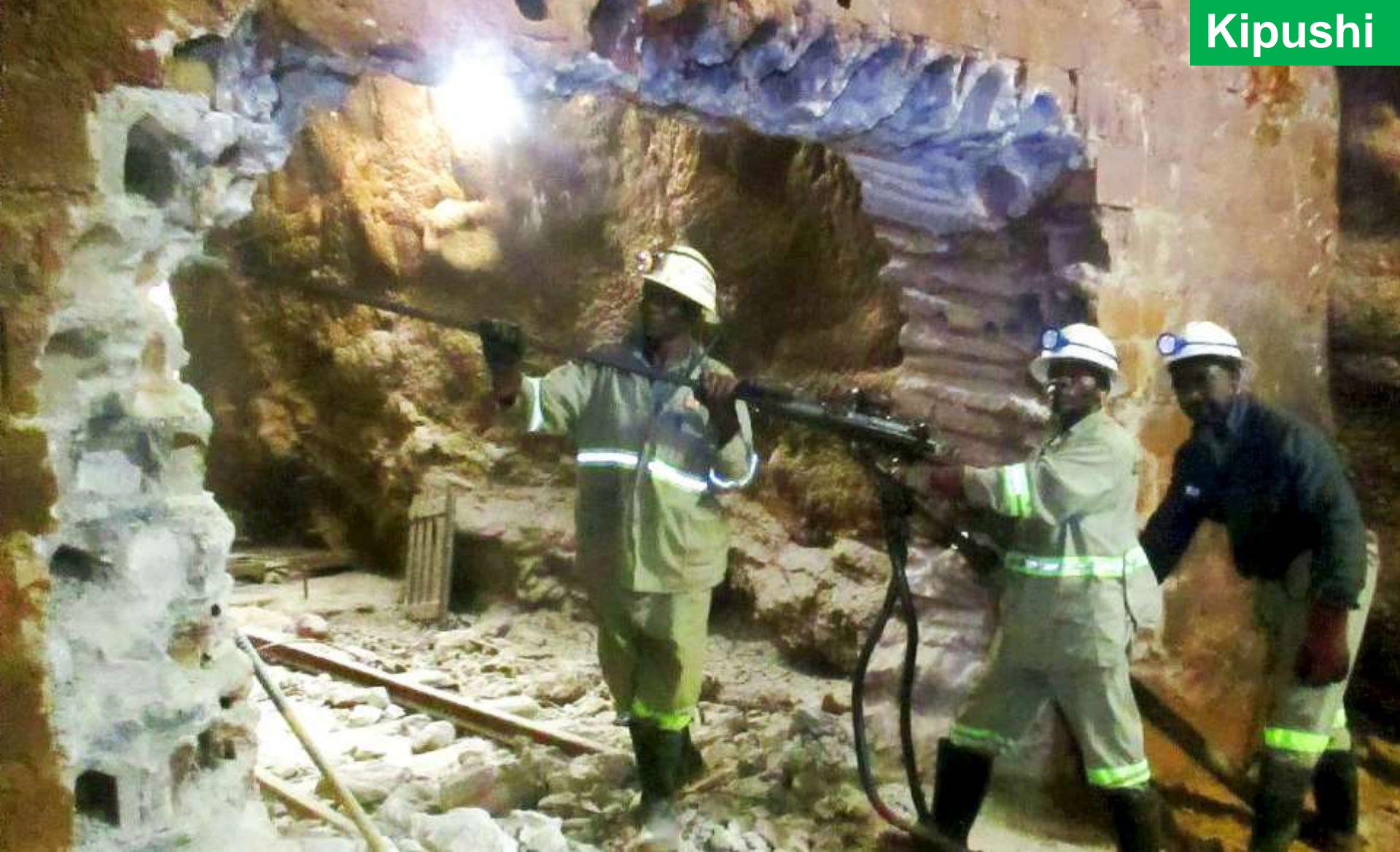
Drilling for installation of an electrical substation at the 1,150-metre level of Shaft 5.
