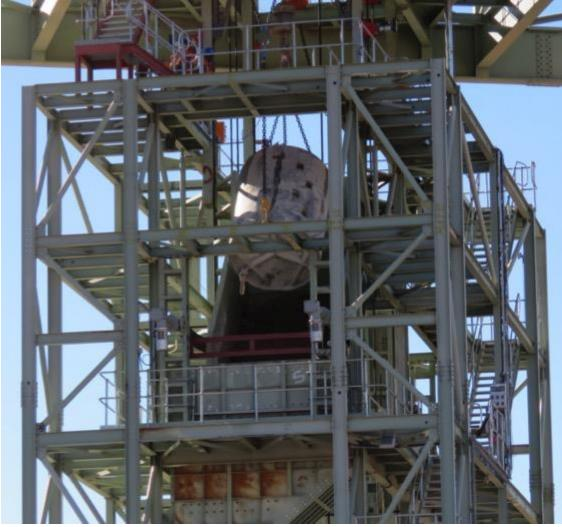
Kibble bucket (left) that is used to remove broken rock from the bottom of Shaft 1 in the ongoing sinking work.
