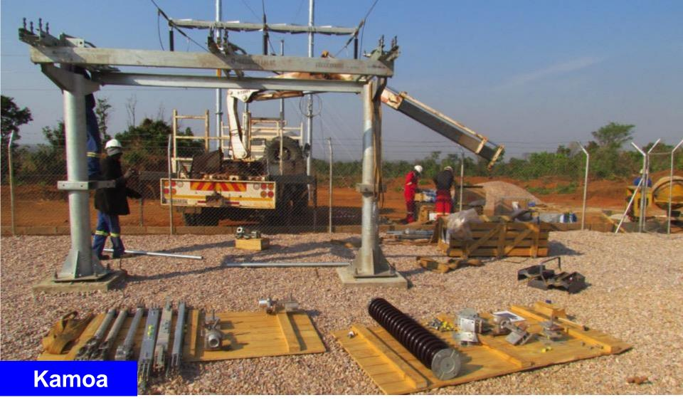
Construction of 120-kilovolt power lines linking the Kamoa site to the national electricity grid is nearing completion.
