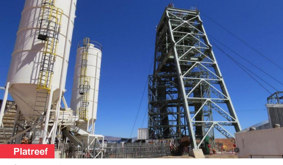
Silos used for storing concrete-making materials adjacent to Shaft 1 headframe.
