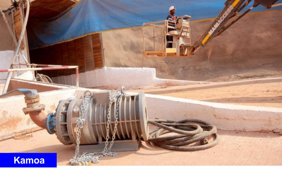
Storm-water pump being prepared for installation at the Kamoa box cut as part of the ongoing development of the twin declines.
