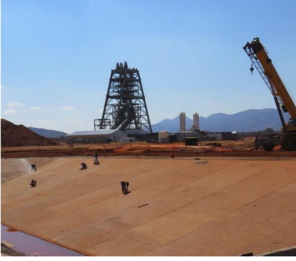
Sealing of concrete joints in storm-water collection ponds at Platreef.
