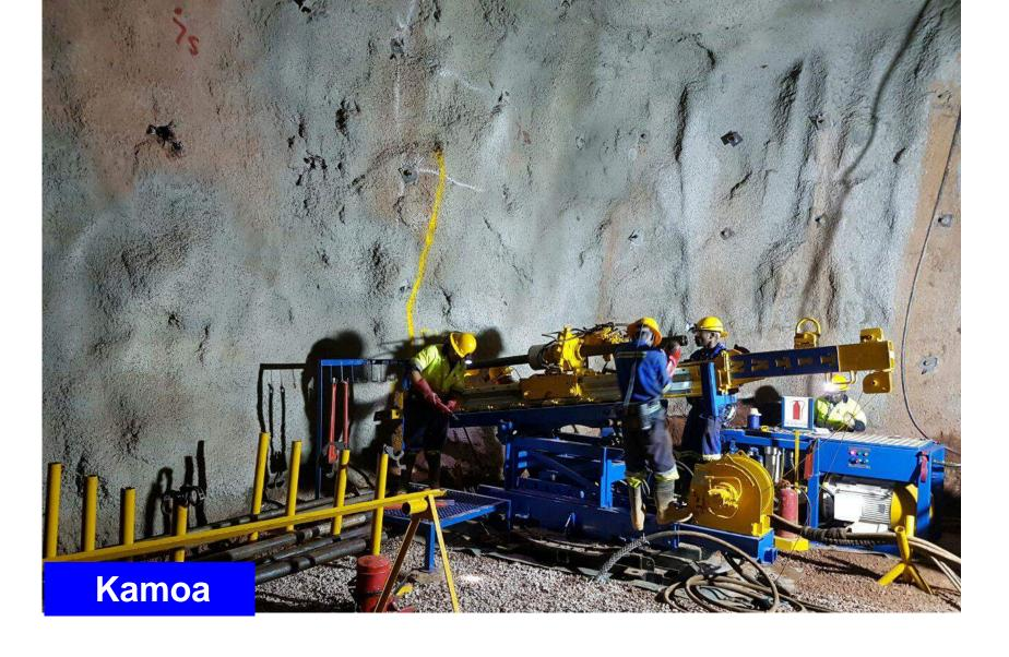
Cover drilling to test water and ground conditions at one of the two declines at Kansoko Sud.
