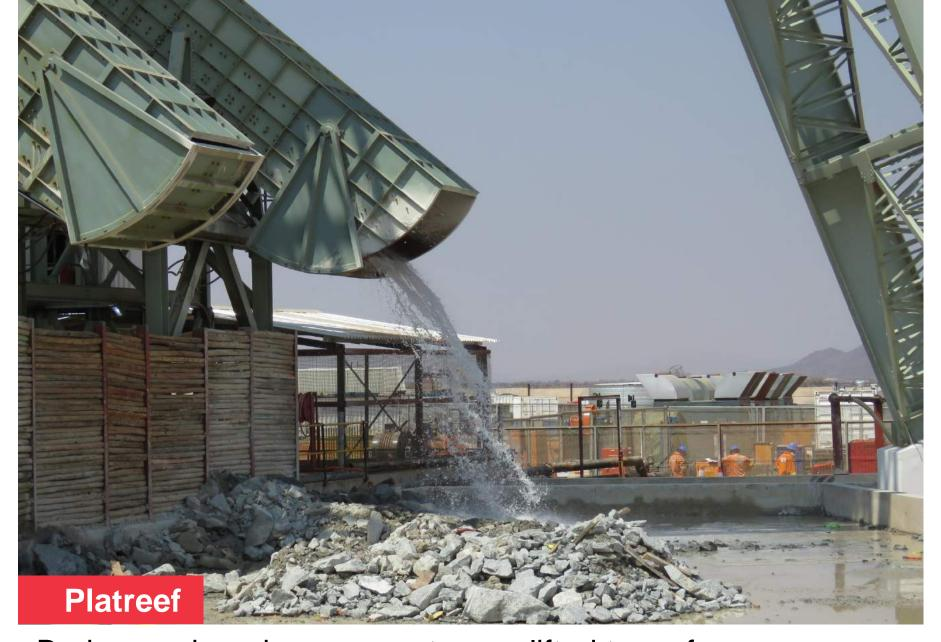
Broken rock and excess water are lifted to surface from the bottom of Shaft 1 during shaft-sinking operations.
