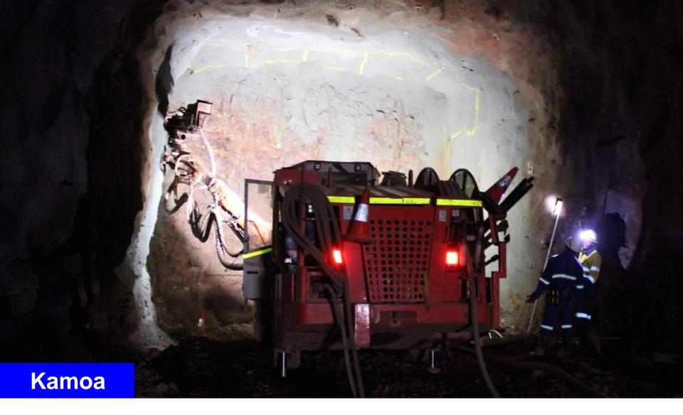
Jumbo drill completing holes for another blast in the ongoing excavation of the declines for the Kansoko Sud mine.
