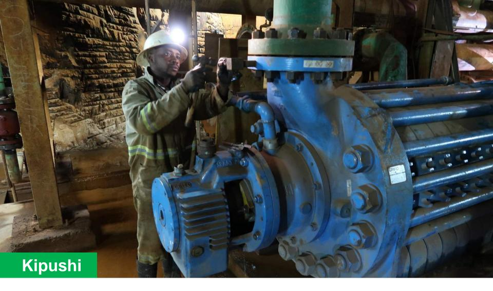
Maintenance of the new Grifo pump at the 1,200-metre-level pumping station.
