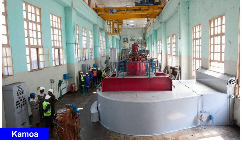
Reconditioned crane and new alternator at the Mwadingusha hydropower plant.
