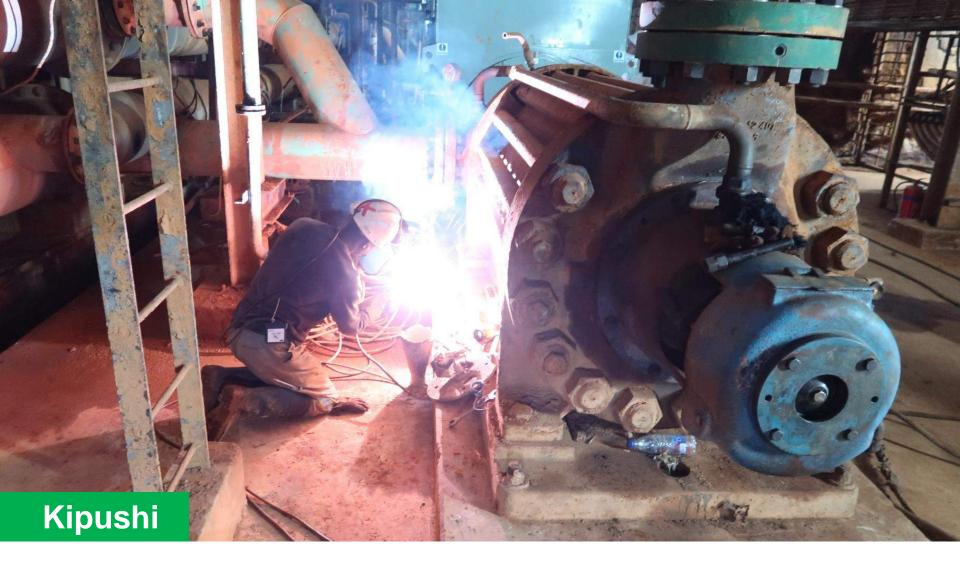
Welding pipe connections for a Sulzer pump at the 1,200-metre-level pumping station.
