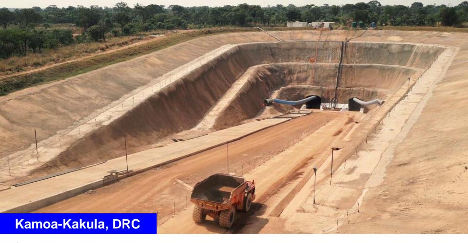
Surface box cut showing entrance to the twin declines being constructed to provide underground mining access to the Kamoa-Kakula Copper Project's initial high-grade Kansoko Mine.
