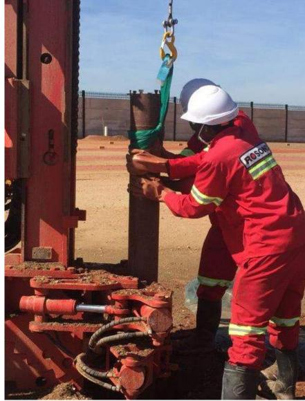
Preparing and installing casing at the excavation site for Platreef's Shaft 2 box cut. The early-works construction for Shaft 2 is expected to take approximately 12 months and cost approximately R70 million (US\$5.5 million).
