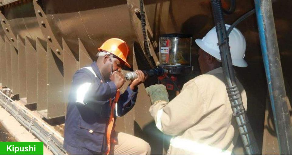
Weekly maintenance of the new, twin, high-volume ventilation fans being commissioned on surface at Shaft 4. These will provide fresh air to the Kipushi Mine's underground workings.
