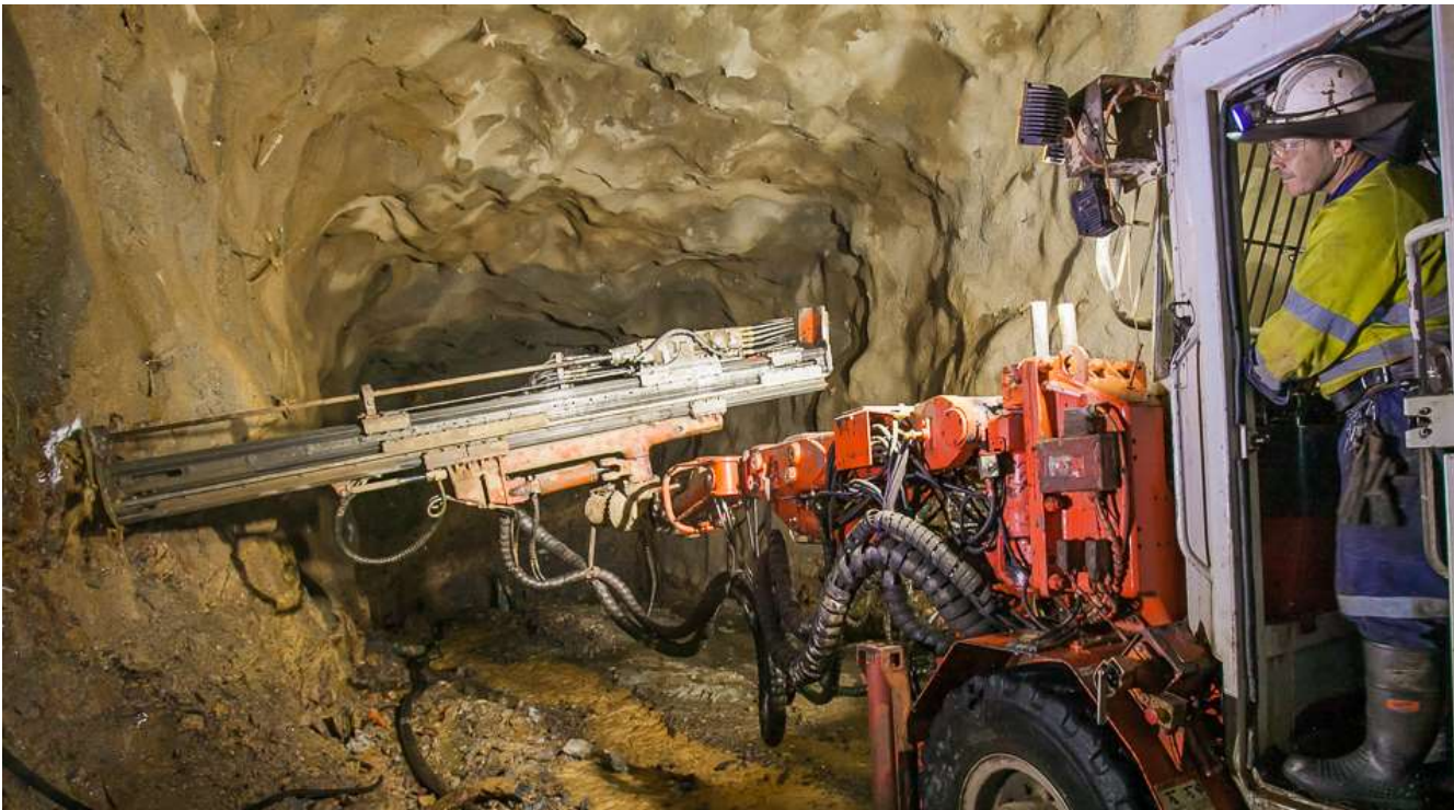
Figure 10: Operating the underground drill rig during decline development.
