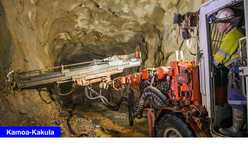
Ongoing construction of access declines for the Kamoa-Kakula Copper Project's high-grade Kansoko Mine. Underground development has advanced the service and conveyor declines approximately 700 metres toward the mineralized area.
