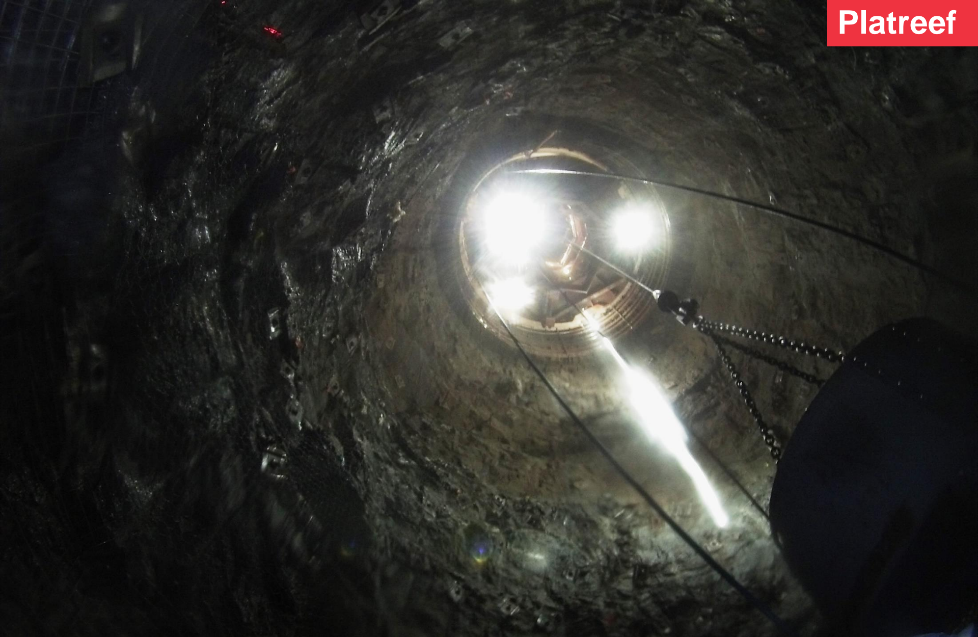
Bucket filled with broken rock from the bottom of Shaft 1 being raised to the surface (view looking up at the pre-sinking stage)
