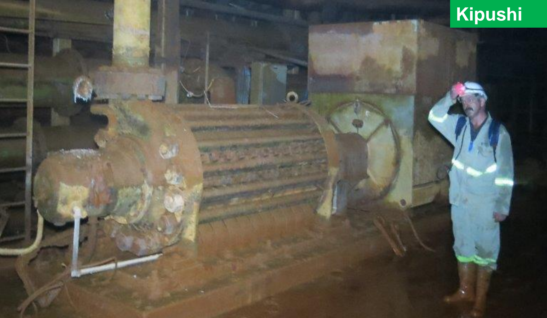
One of five existing high-capacity Sulzer pumps in the main pumping station at the Kipushi Mine's 1,210-metre level that were recovered in December 2015 following a successful dewatering program. The pumps, which had been submerged and disabled since the mine flooded in early 2011, will be upgraded and returned to service later this year.
