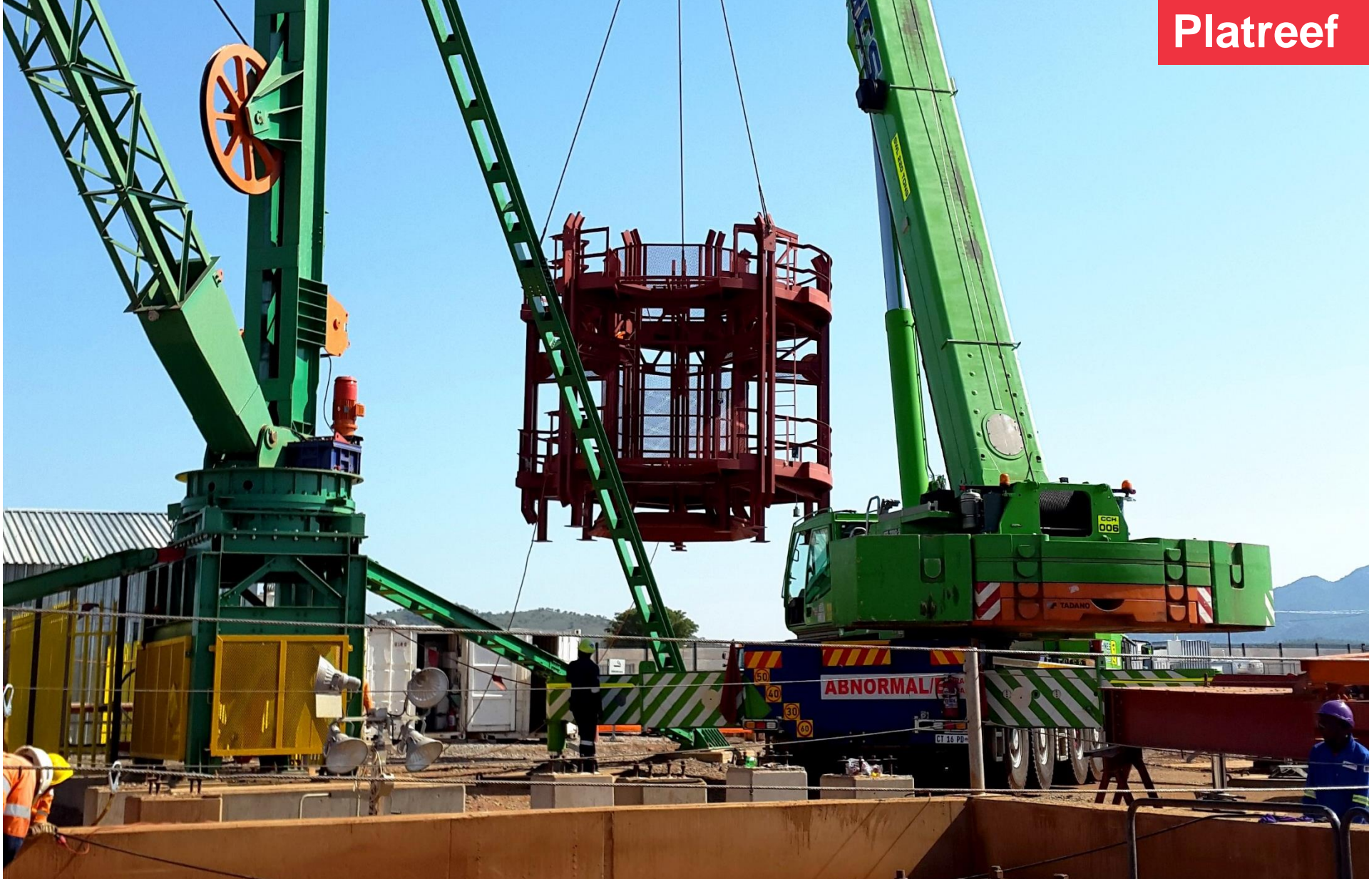
Installation of the working platform (stage) for the pre-sinking phase at Shaft 1
