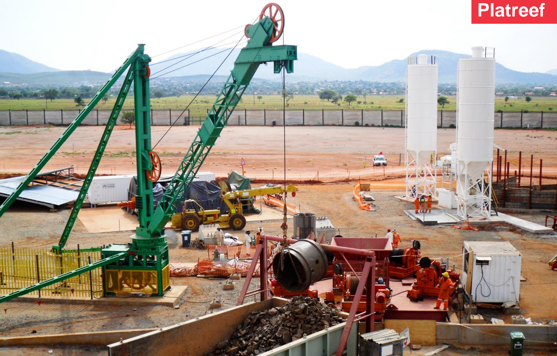
Unloading a bucket of broken rock excavated from Shaft 1
