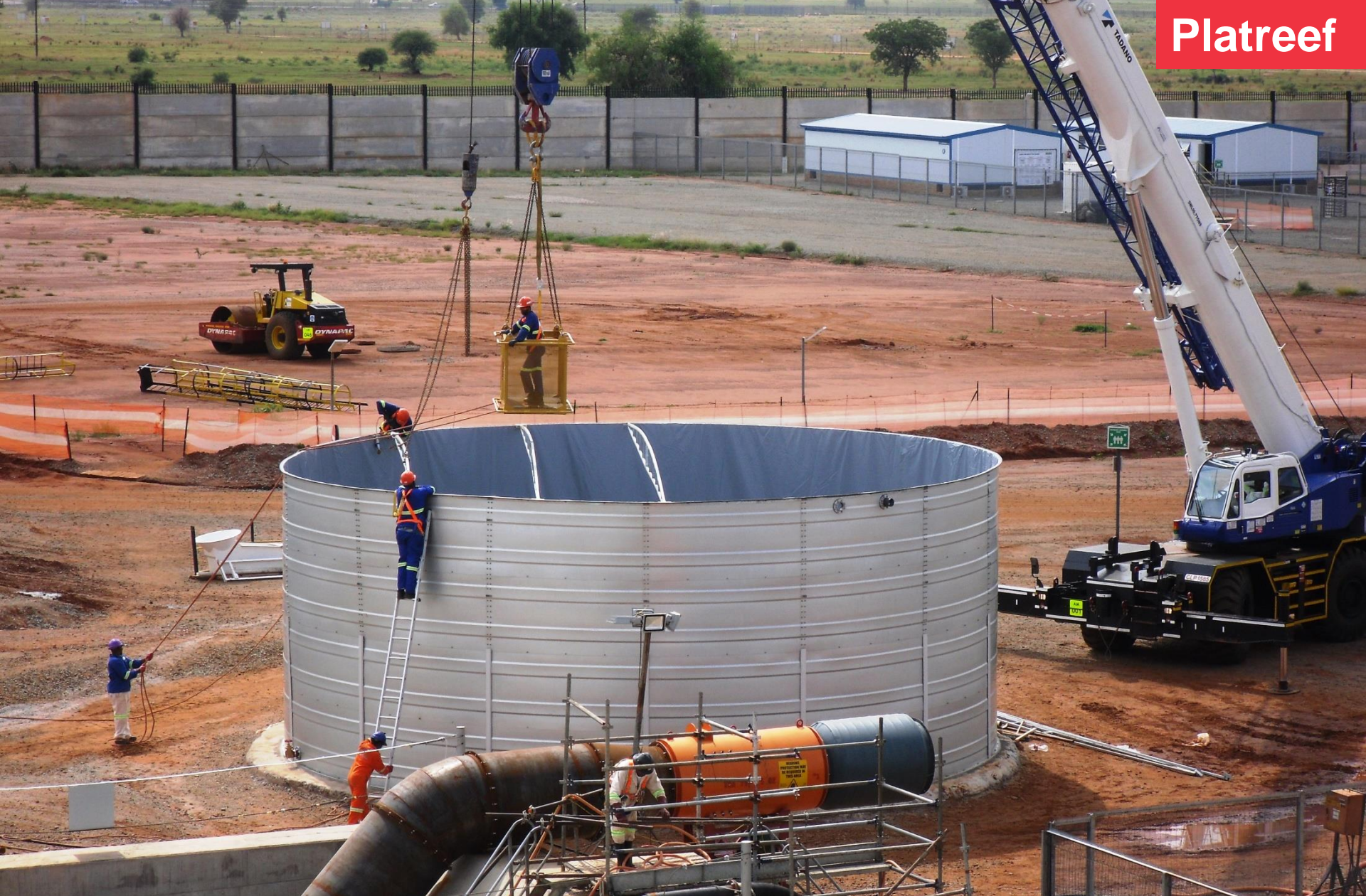
Installation of the Shaft 1 water tank
