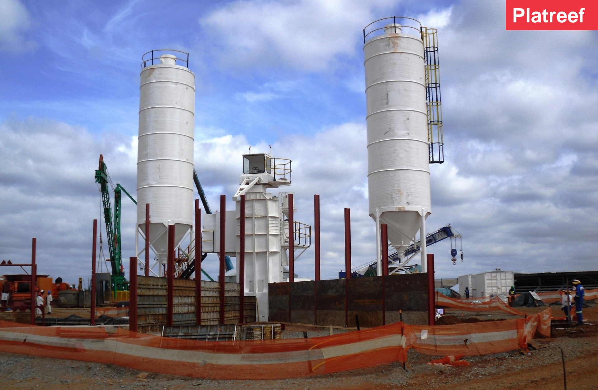
Batch plant, now nearing completion, will provide concrete to line the wall of Shaft 1
