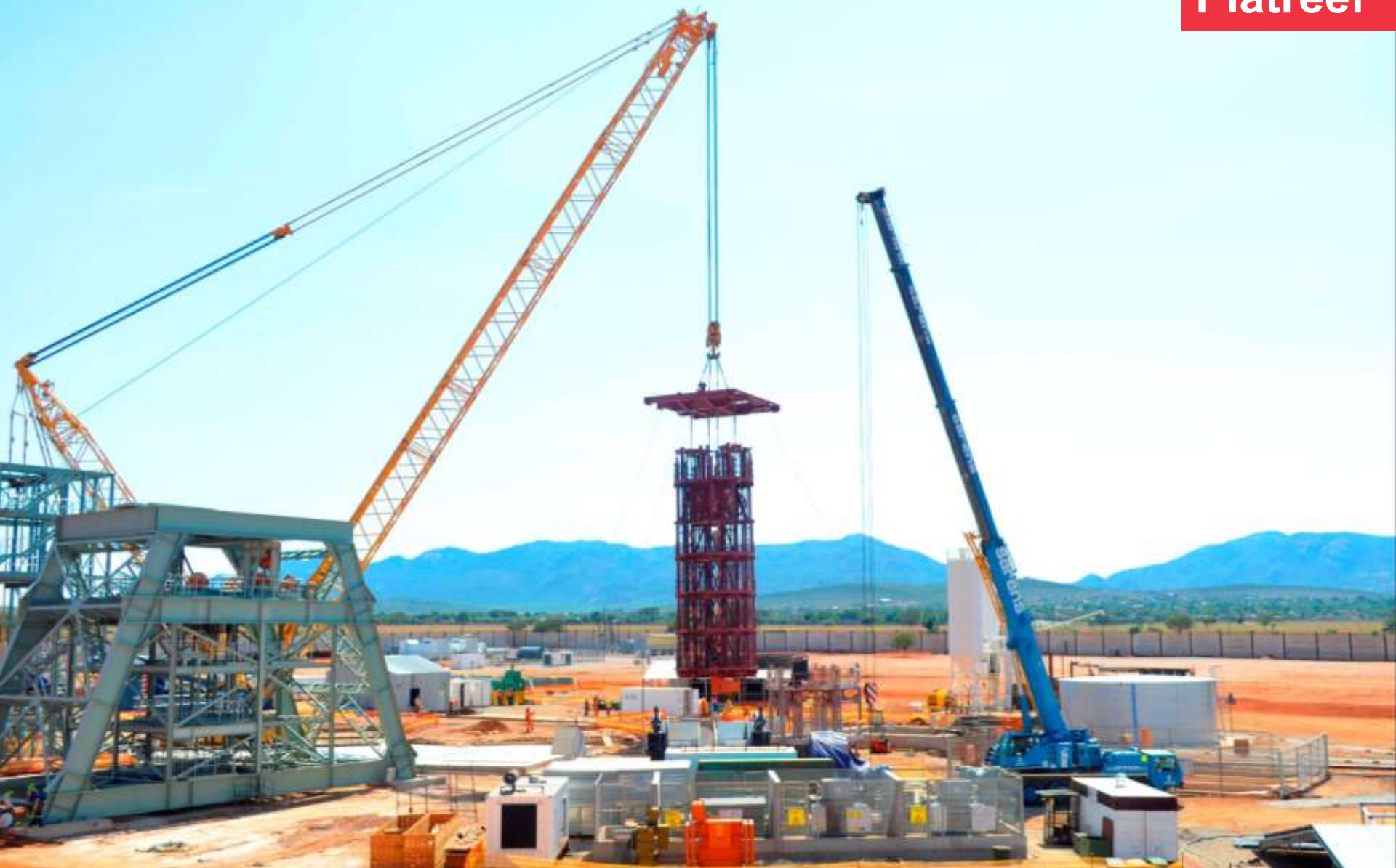
Lowering of the five-deck stage into Shaft 1
