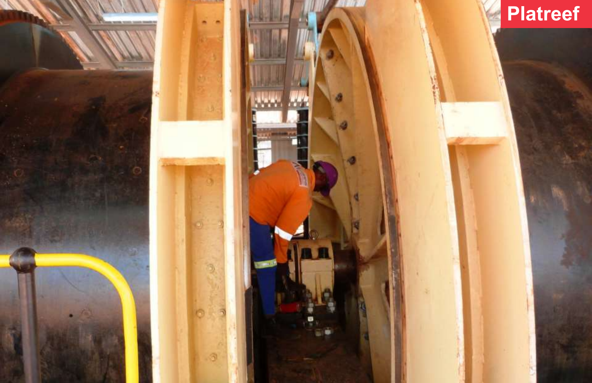
Final mechanical alignment work on the stage winder
