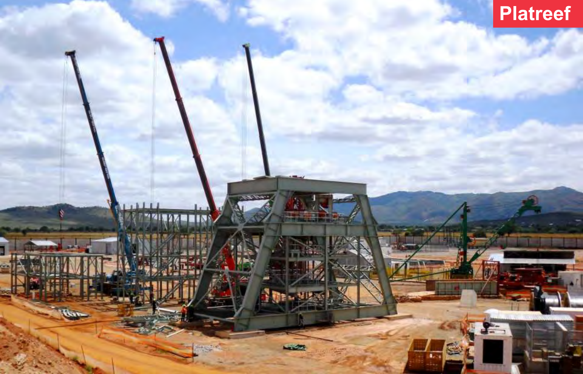
Pre-assembled structural steelwork for Shaft 1 head gear and tower
