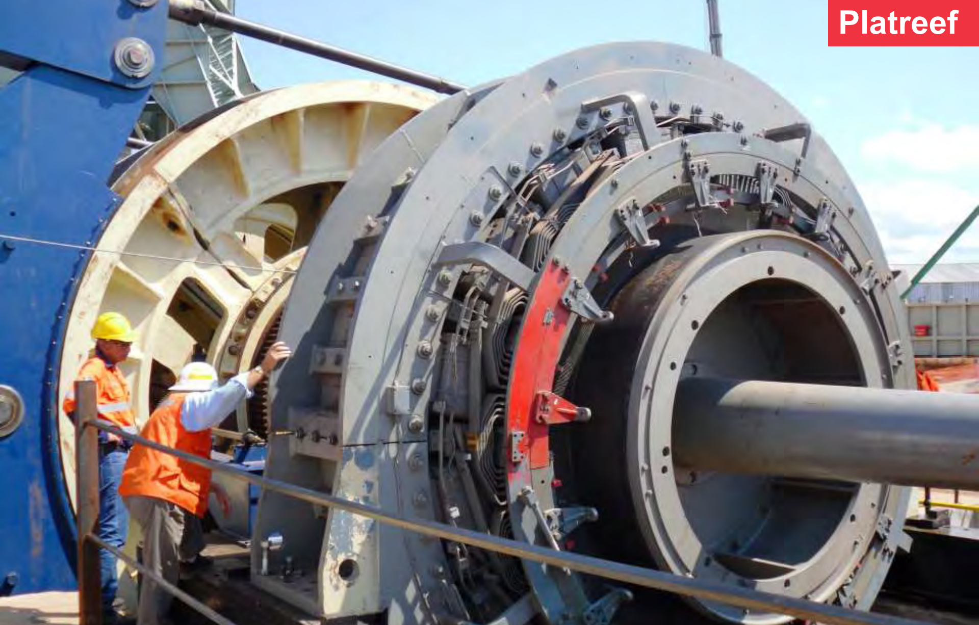
Installation of the hoisting winder motor to be used for Shaft 1 sinking operations
