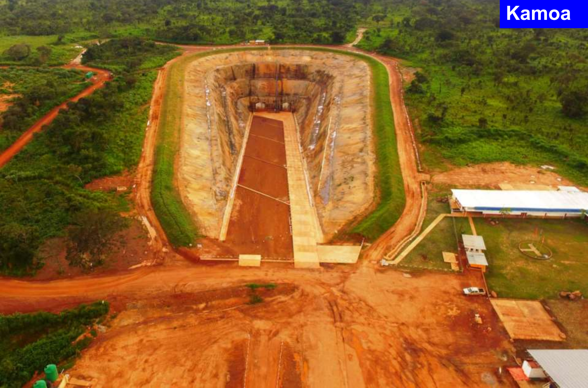
Kamoa box cut, which will provide underground access during the construction and operation of the initial mining area
