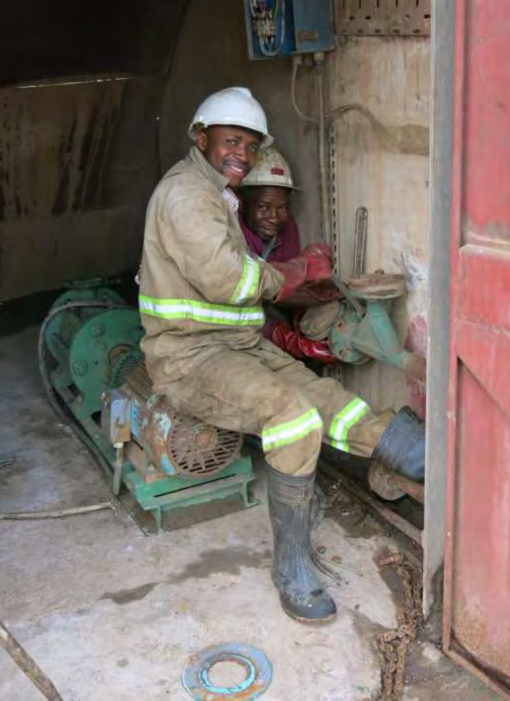
Workers repair Shaft No. 5 water pump
