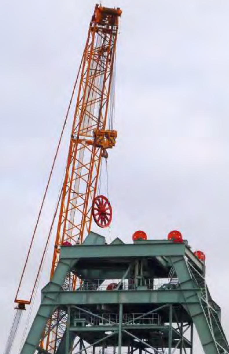
Installation of sheave wheel on top of Shaft 1 head gear
