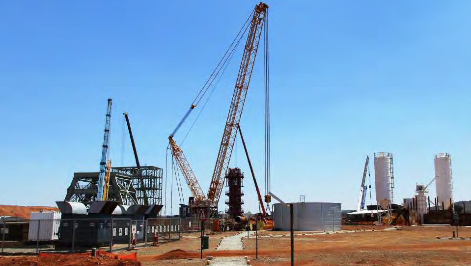
Mine-site work area showing crane – capable of lifting 800 tons – used in the erection of the head gear for Shaft 1
