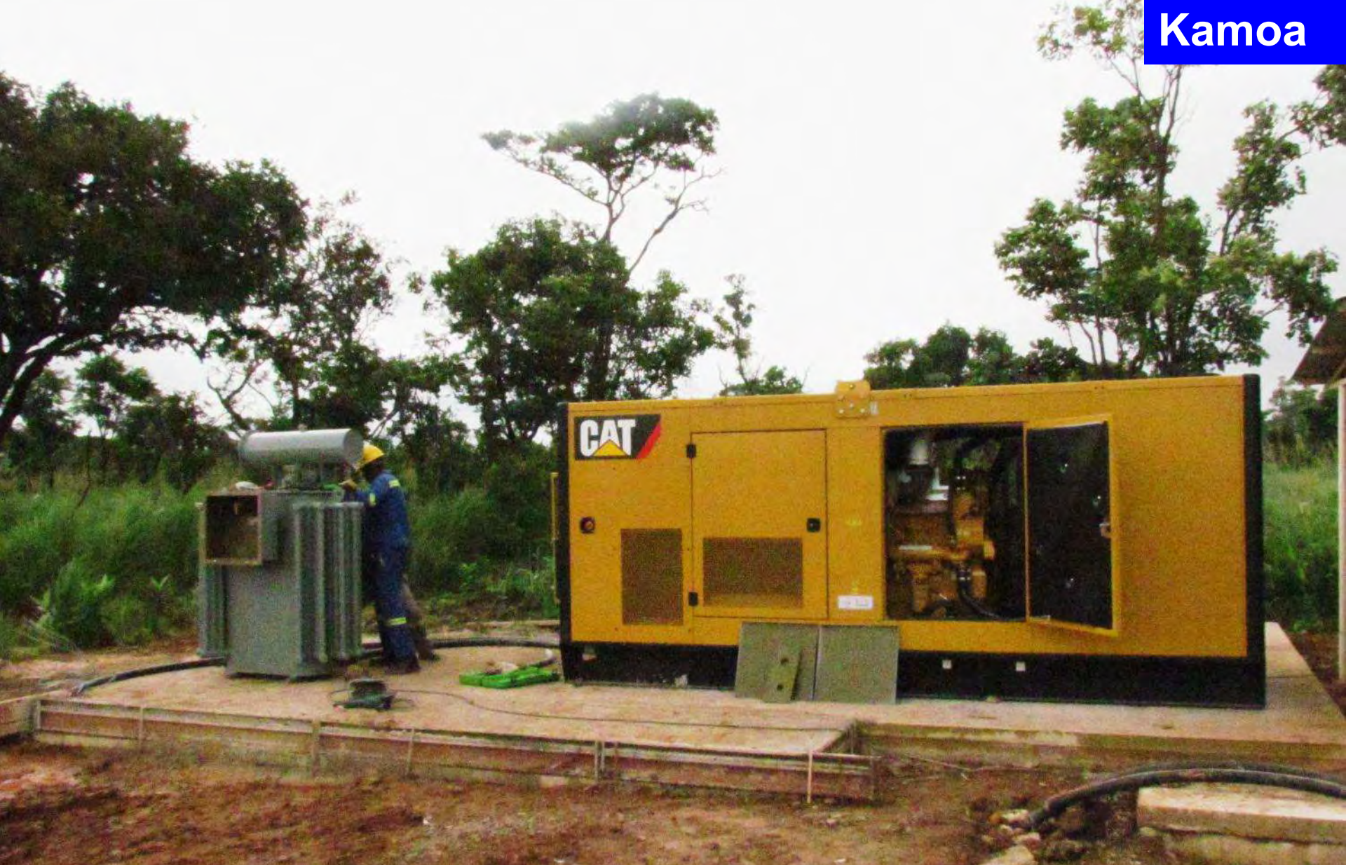
Installation of the new 400kva generator at the Kamoa box cut
