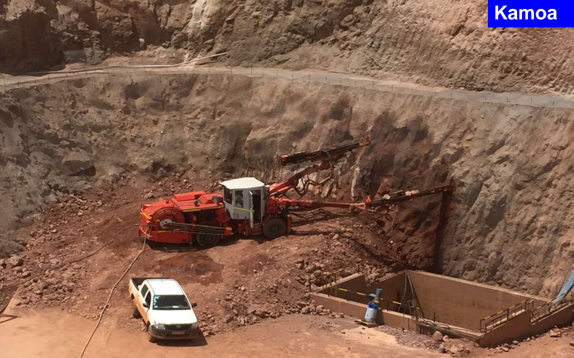
Twin-boom rig drilling 3-metre rebar holes above the site for one of the Kamoa declines.
