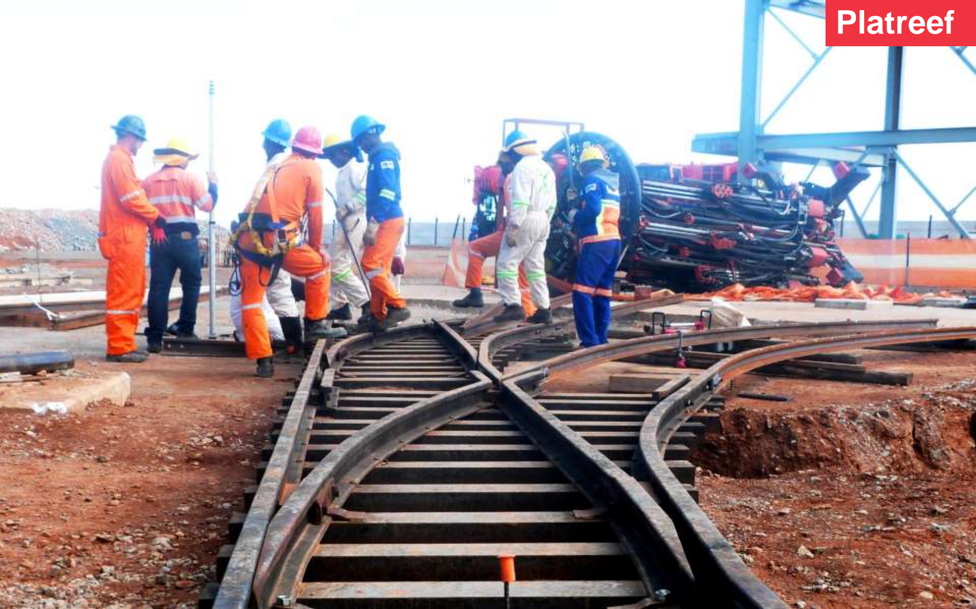
Track installation at Shaft 1 for the transportation of the jumbo drill.
