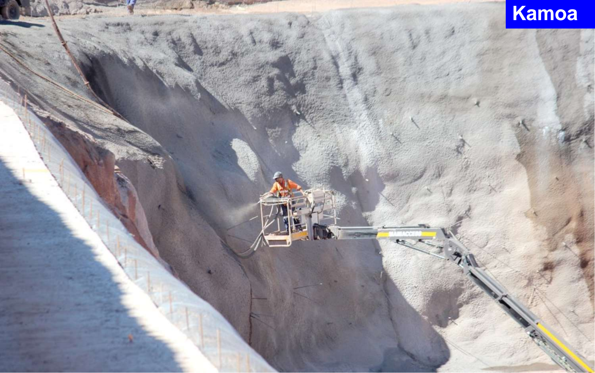
Applying shotcrete to the eastern high wall of the Kamoa box cut.
