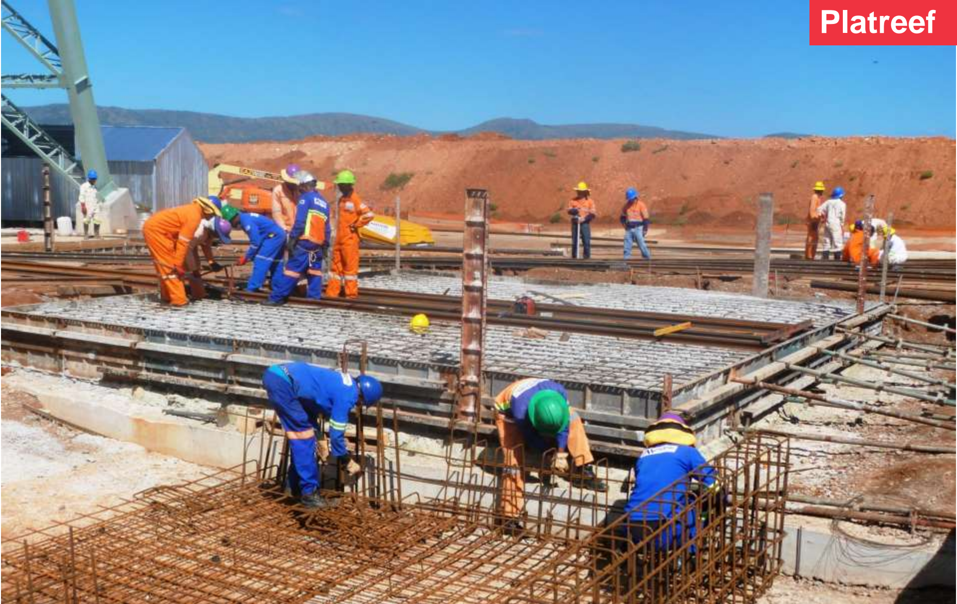
Platform and jumbo-drill pad construction at Shaft 1.
