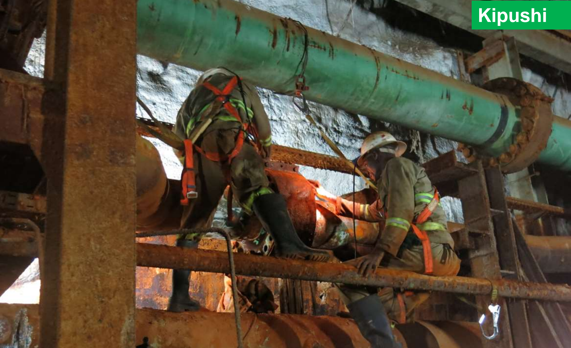
Workers change valves at the 1,200-metre pump station.
