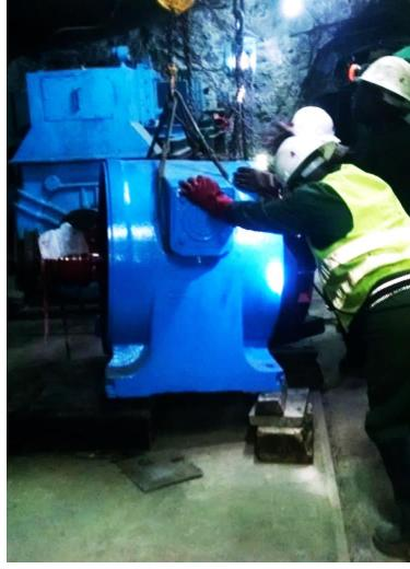
A motor generator is upgraded (left) and re-installed underground (right).
