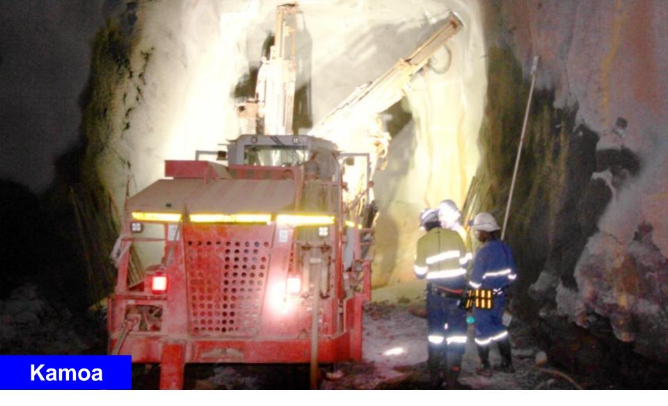
Jumbo drill completing holes for another blast in the ongoing excavation of the declines.
