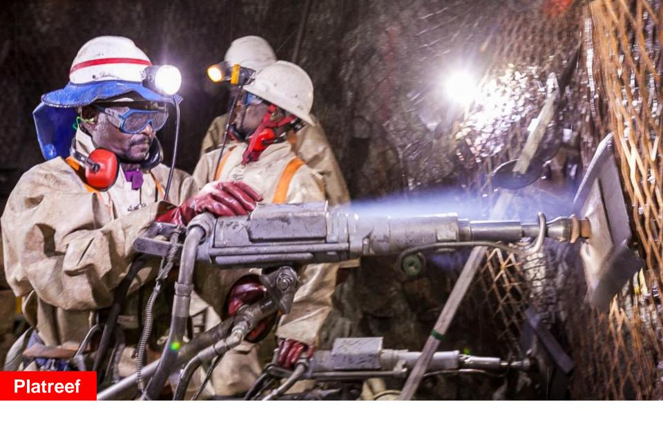
Shaft workers drilling holes for installation of sidewall support units in Shaft 1.
