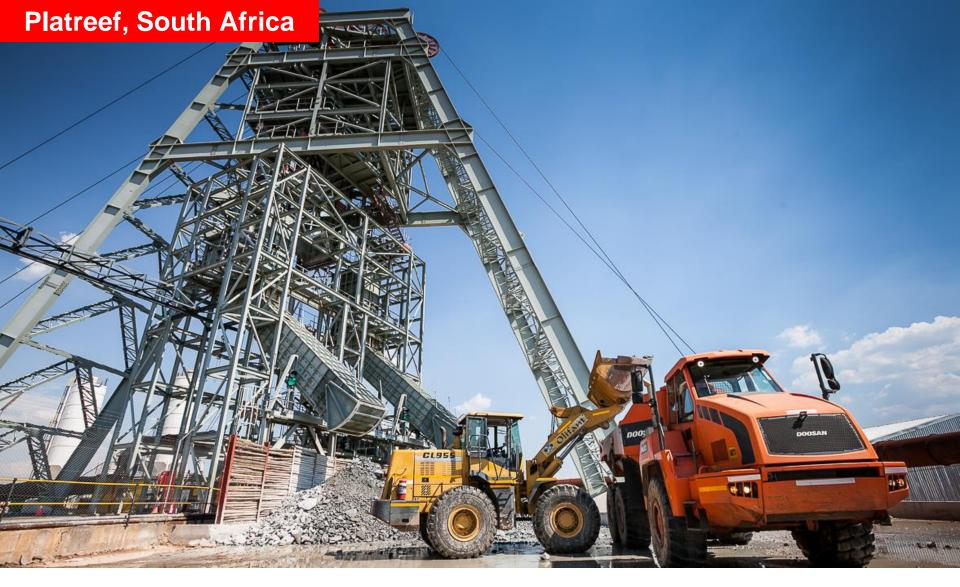
Platreef Project's Shaft 1 head gear and infrastructure, showing excavated rock from shaft sinking being removed from site. Shaft 1 had been sunk to a depth of 204 metres below surface on January 30, 2017.
