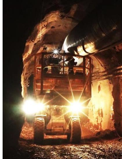
Twin-boom drill rig (left) and utility vehicle (right) used to develop and construct the declines.
