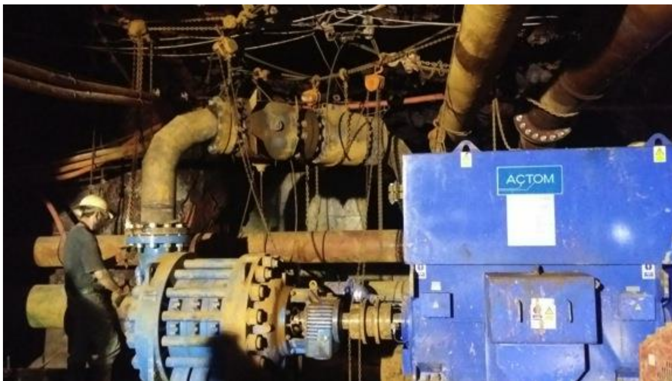
Figure 12: Installation of new Grifo pump at 1,112-metre pump station.
