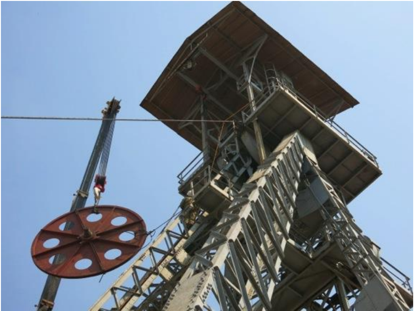
Figure 13: Replacing sheave wheel on Shaft #2 headframe.
