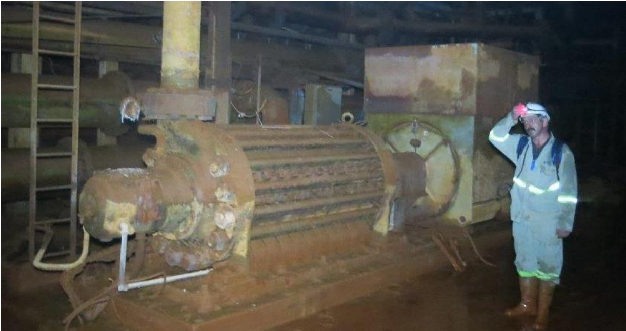
Figure 8: One of five existing high-capacity Sulzer pumps in the main pumping station that will be refurbished.
