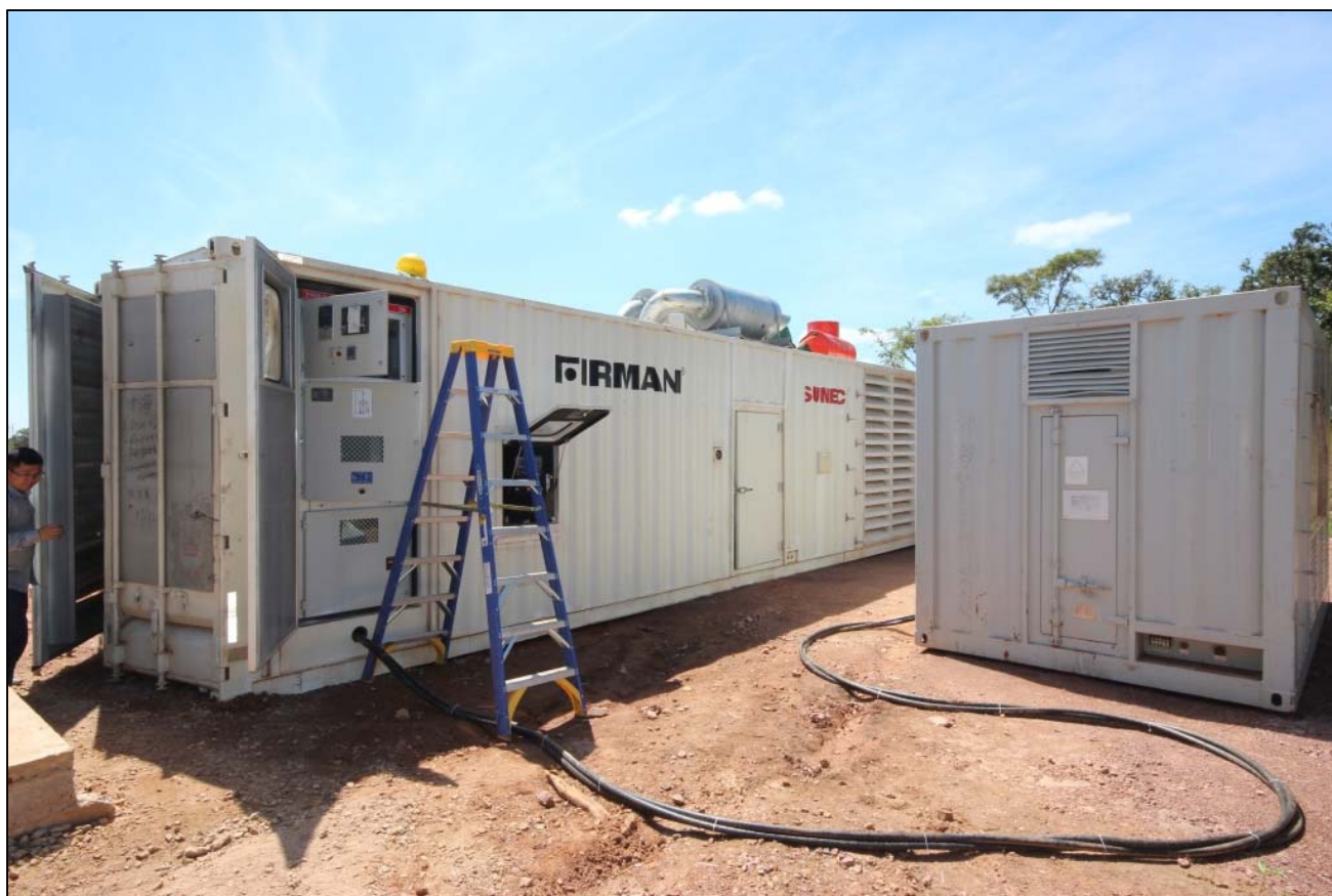
Figure 14: Sumec 2-MW generator being commissioned.
