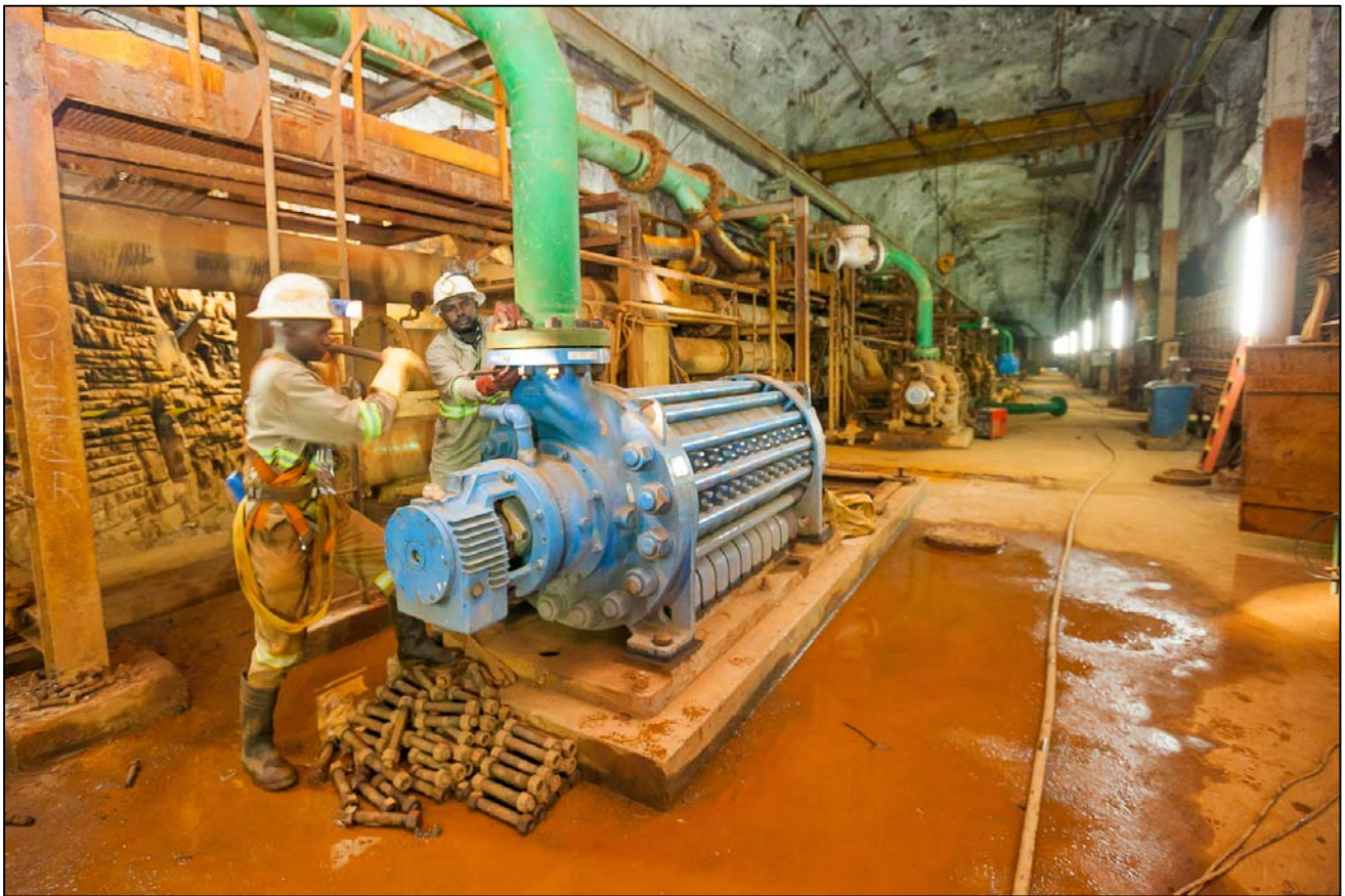
Figure 6: Main pump station in Shaft 5 at 1,200-metre-level with installation of Grifo centrifugal pump.
