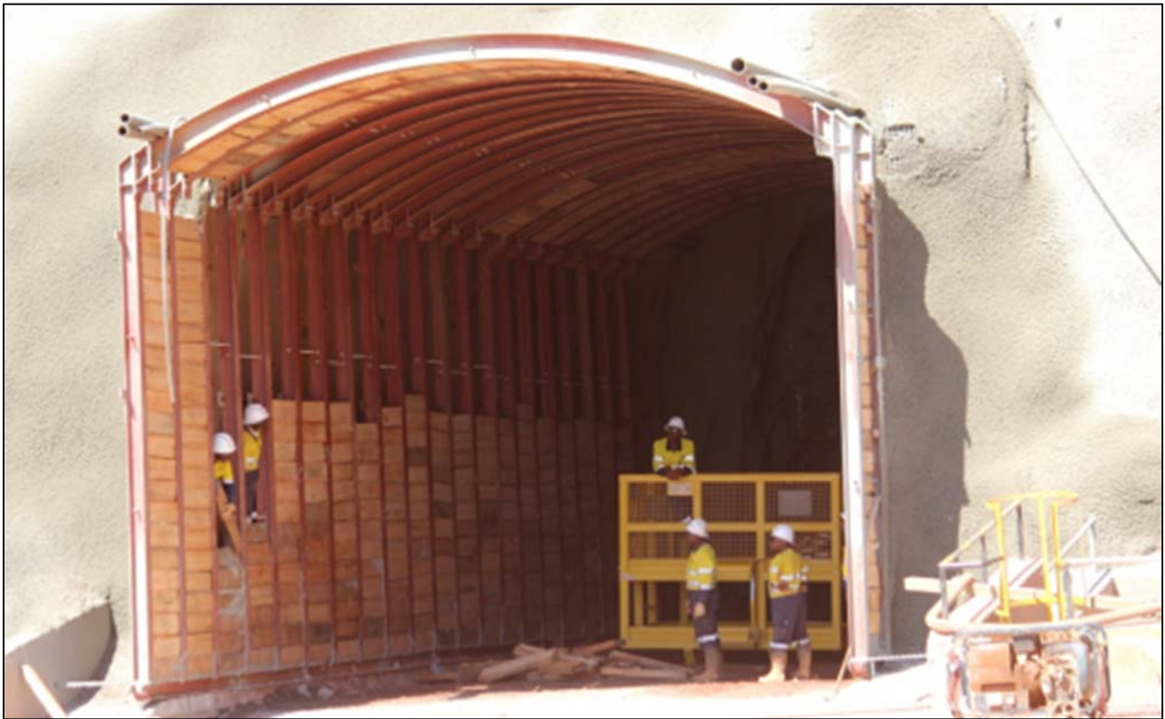
Figure 11: Conveyor decline sets.
