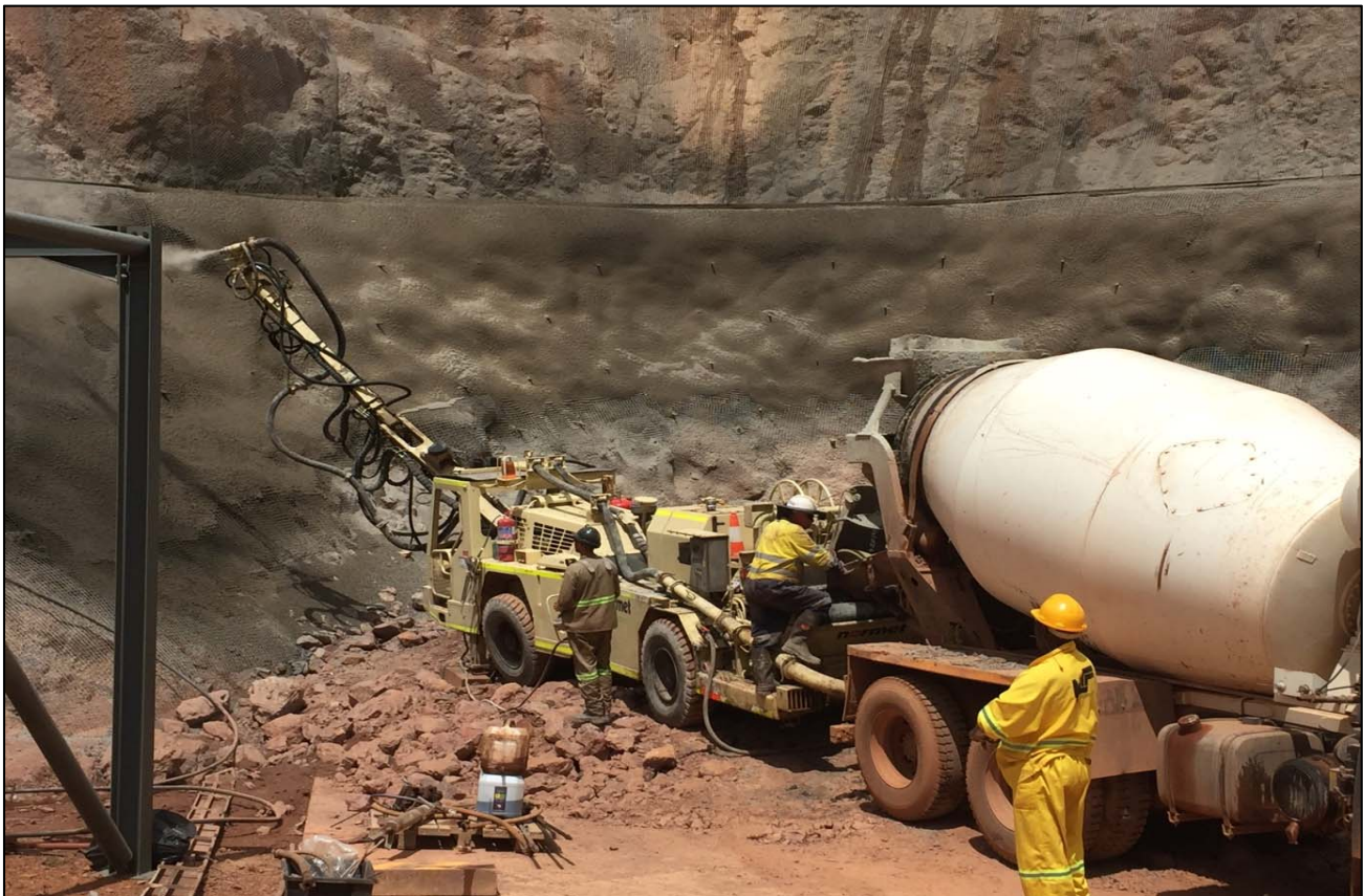
Figure 16: Shotcrete application on the bottom bench.
