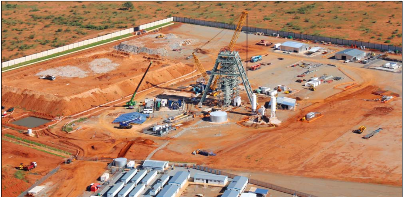
Figure 4: Aerial view of Shaft 1 headgear and related surface works.
