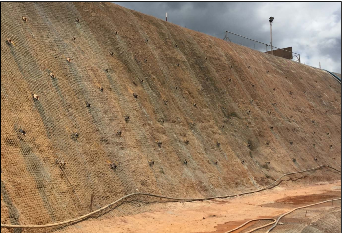
Figure 15: Installed mesh and three-metre rebar bolts.
