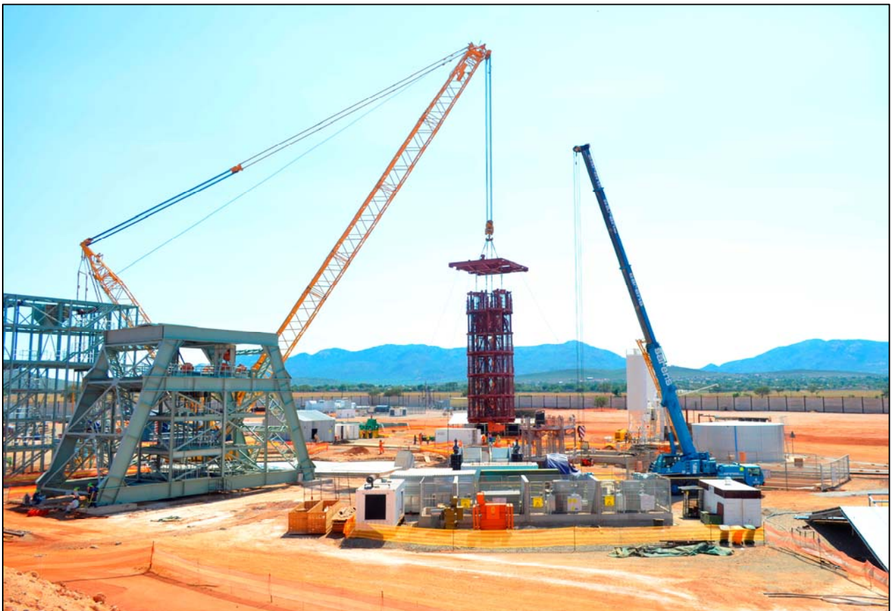
Figure 2: Lowering of the five-deck stage and bank steelwork into Shaft 1.
