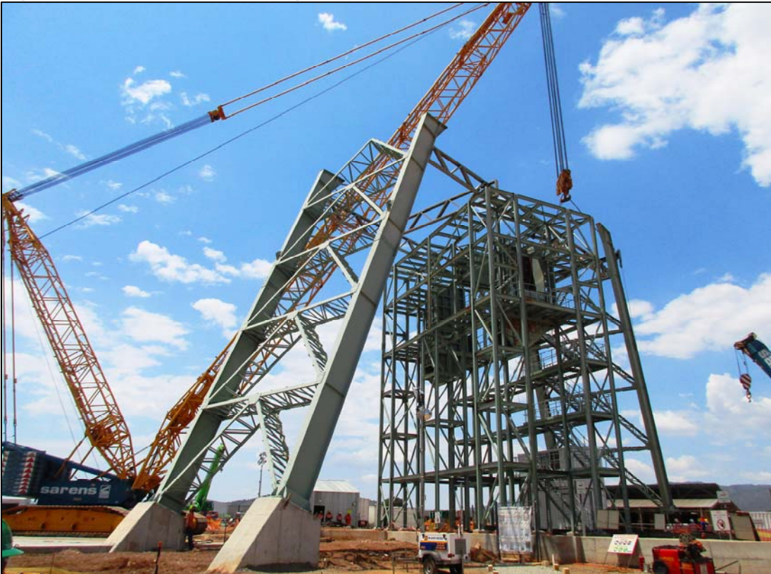
Figure 3: Construction of headgear for main sinking operations.
