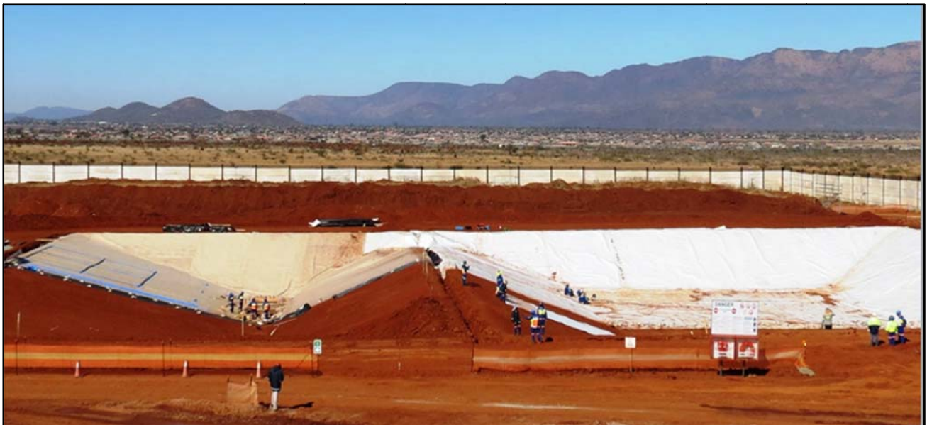
Figure 7: Construction of the lined storm-water pond.
