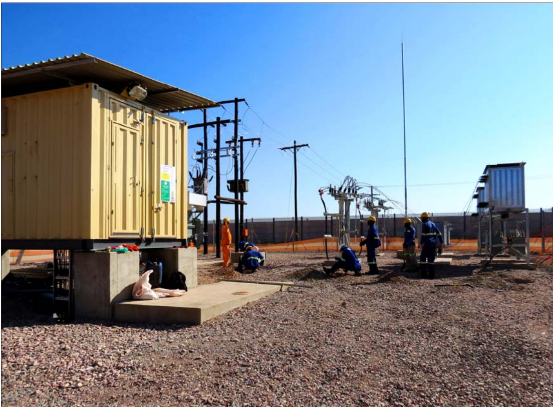
Figure 5: 5MVA sub-station and lines to deliver Eskom power.
