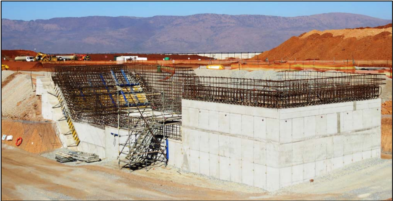
Figure 3: Shaft 1 collar and ventilation plenum construction, July 2015.
