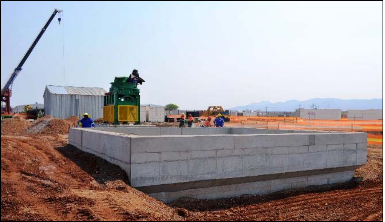
Figure 7: Initial sinking activities at Shaft 1 bottom.
