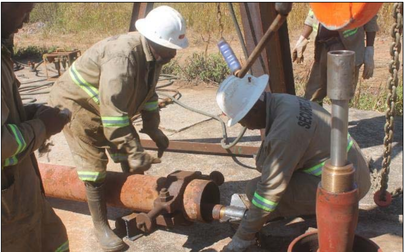
Figure 14: Refurbishment of a borehole pump in the potable water wellfield supplying all of Kipushi municipality.
