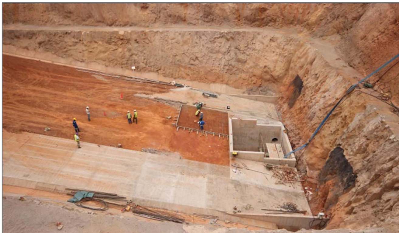
Figure 2: Box-cut civil works in progress on the sump and roadway.
