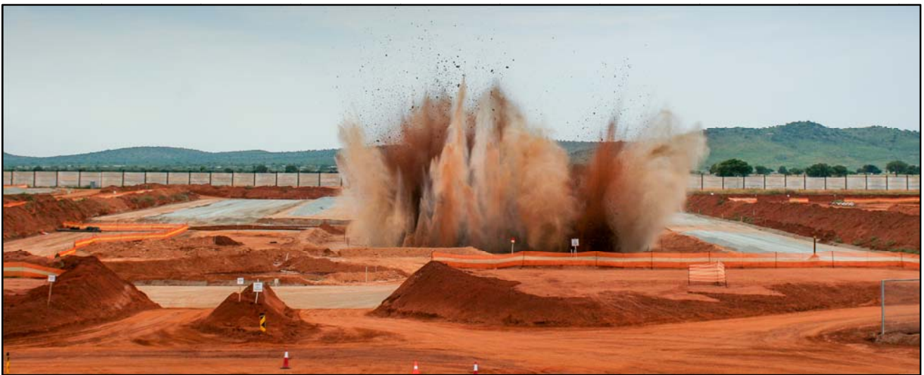
Figure 5: First blast at Shaft 1 box cut.
