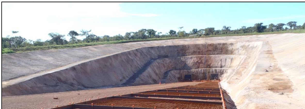
Figure 2: Completed box cut with access roadway under construction.
