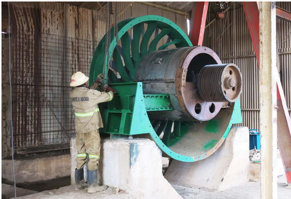
Figure 12: Ventilation shaft fan refurbishment.
