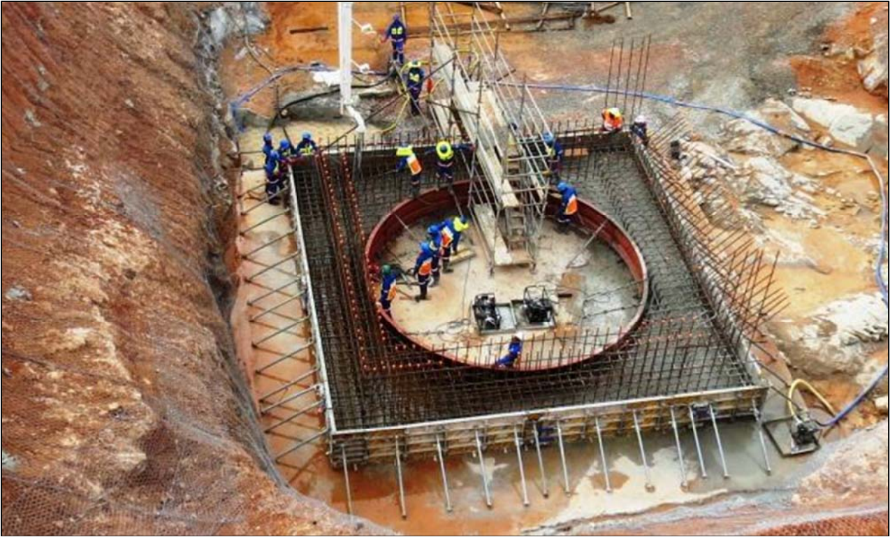
Figure 5: Construction of Shaft 1 collar, May 8, 2015.
