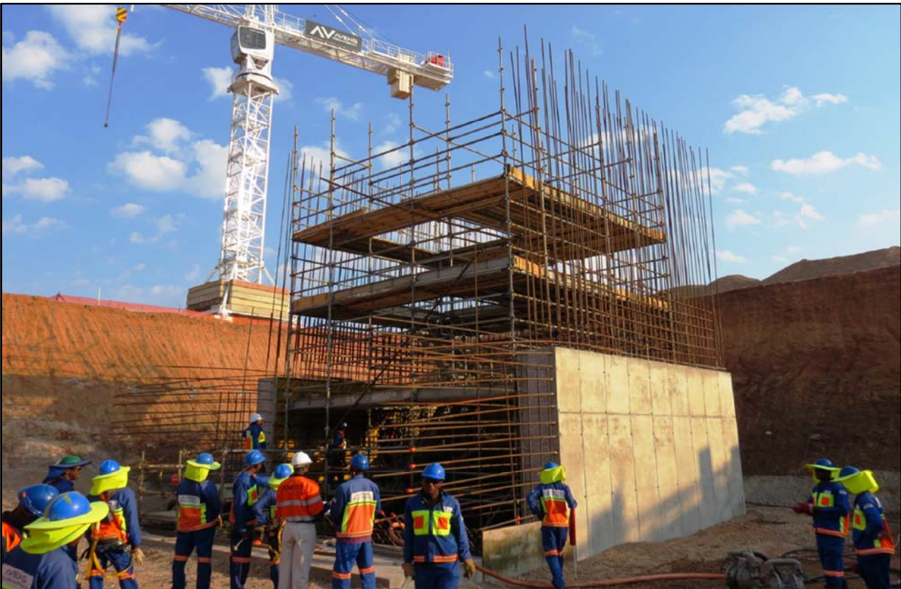
Figure 5: Construction of Shaft 1 collar, May 8, 2015.
