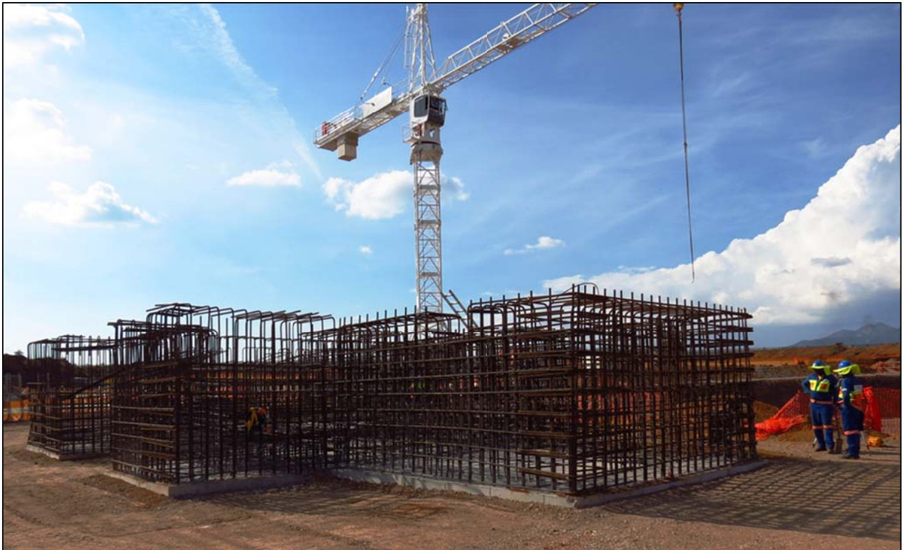
Figure 6: Construction of Shaft 1 kibble winder foundation.
