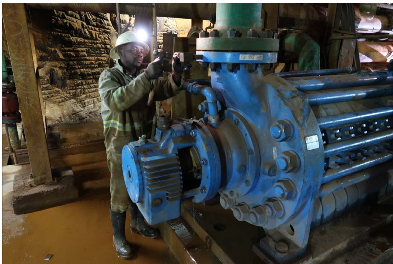
Figure 3: Connecting discharge pipes to one of five pumps on the 1,200-metre-level.
