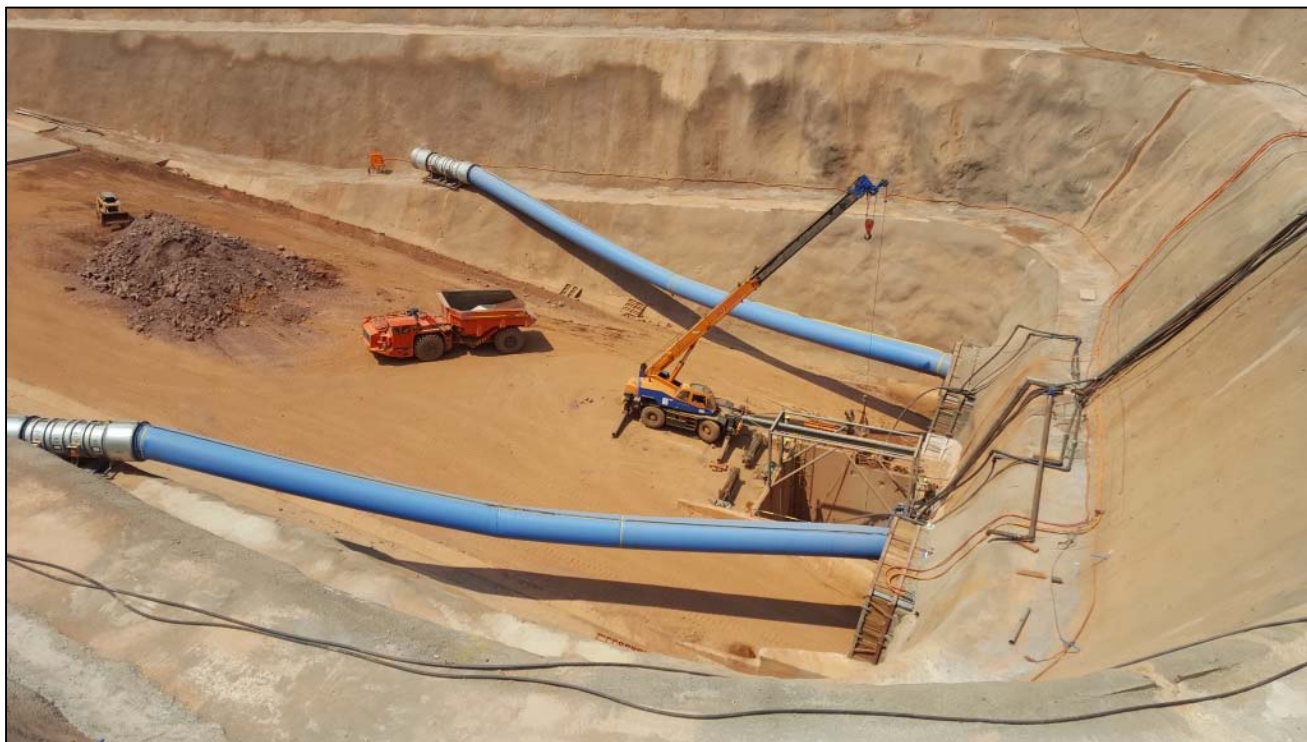
Figure 6: Kansoko box cut sump being cleaned and equipped.
