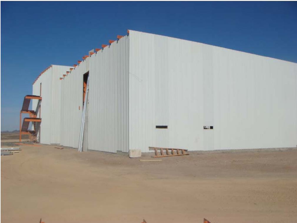
Permanent Camp at Ovoot Tolgoi (windows to be installed shortly)
