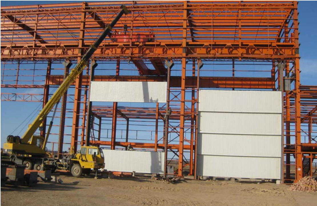
Overhead doors being installed on permanent shop
